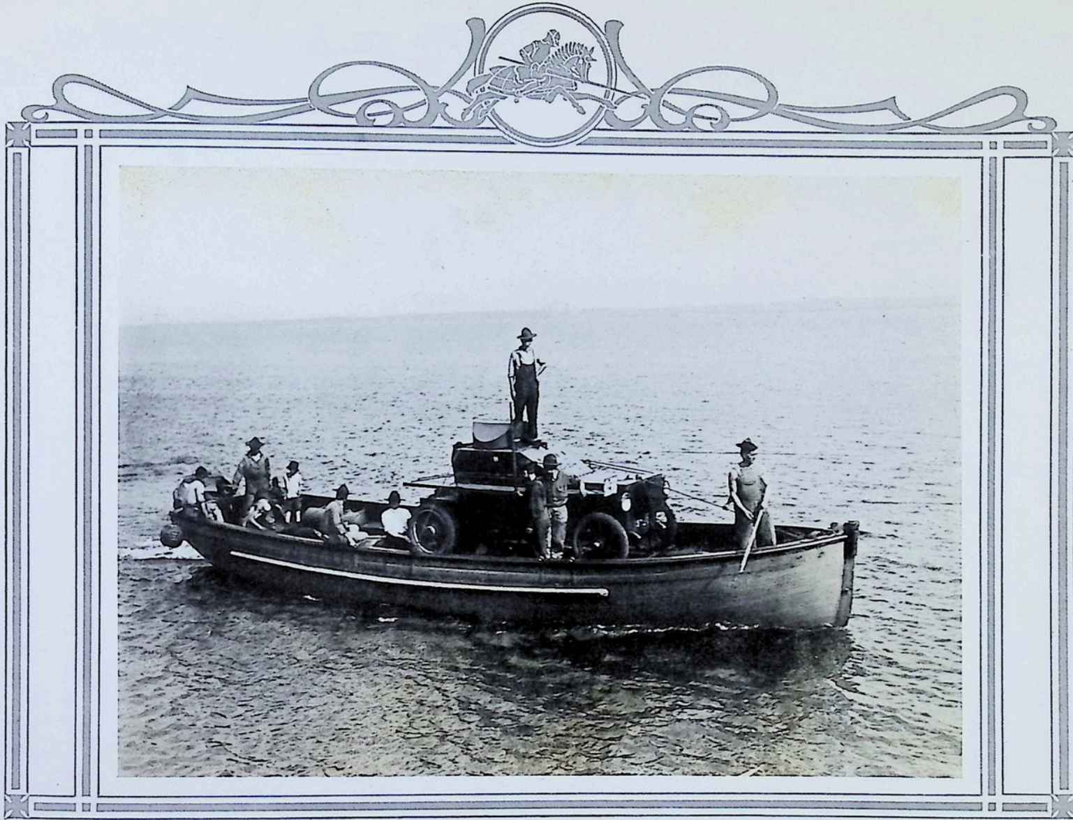
Returning to crane after landing test. Note that the Armored Car converts the motor sailer into an armored boat for covering landing parties.
