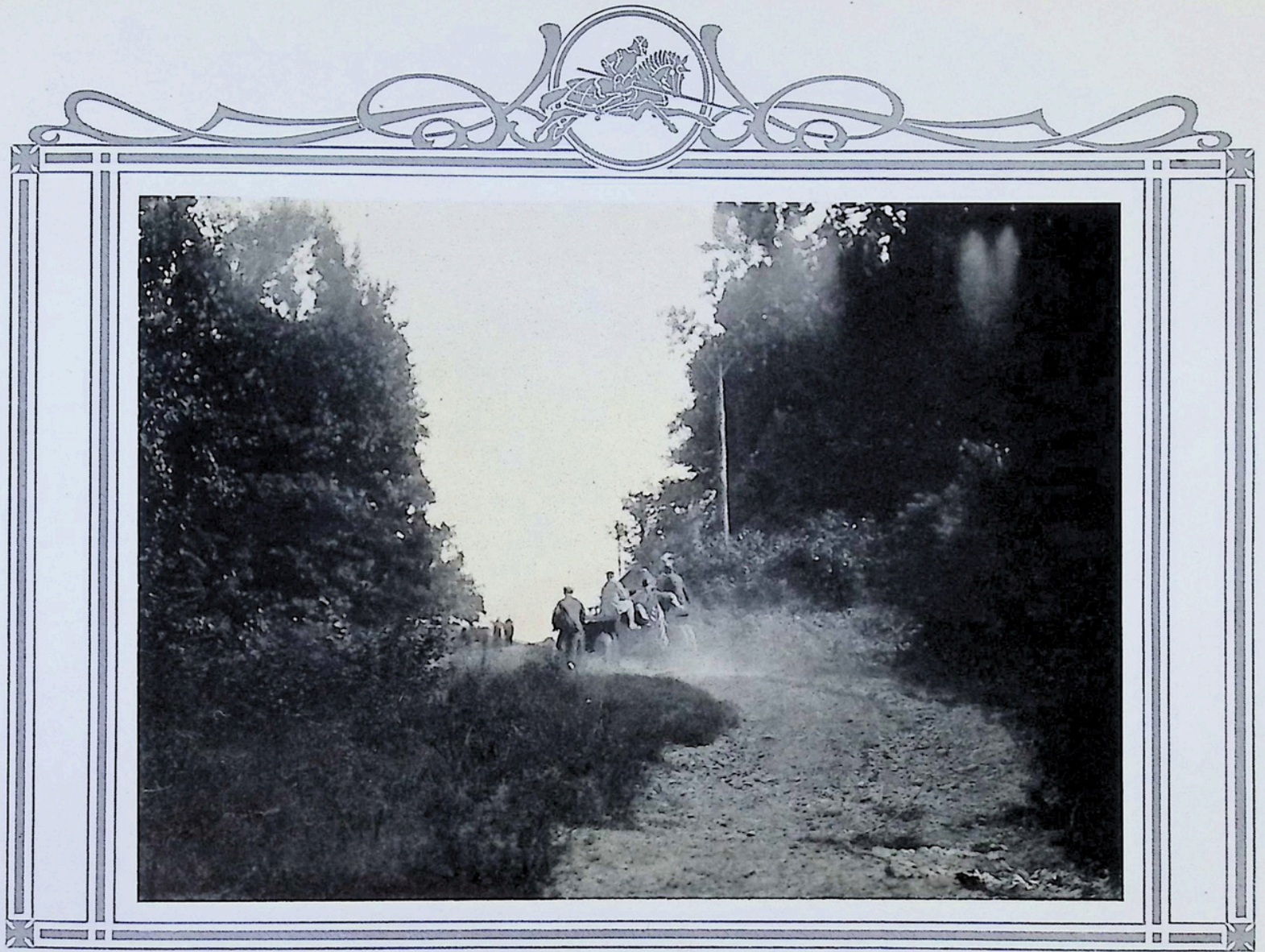
Over summit, Back Hill Road, Fort Myers, Va. Surface of roadway badly cut up by ditches. Traction extremely poor, owing to small cobbles on surface.
