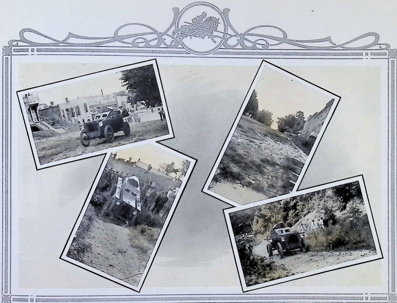
Group of photographs of Washington Test. Upper right-hand picture gives good idea of 35th Street Grade.
