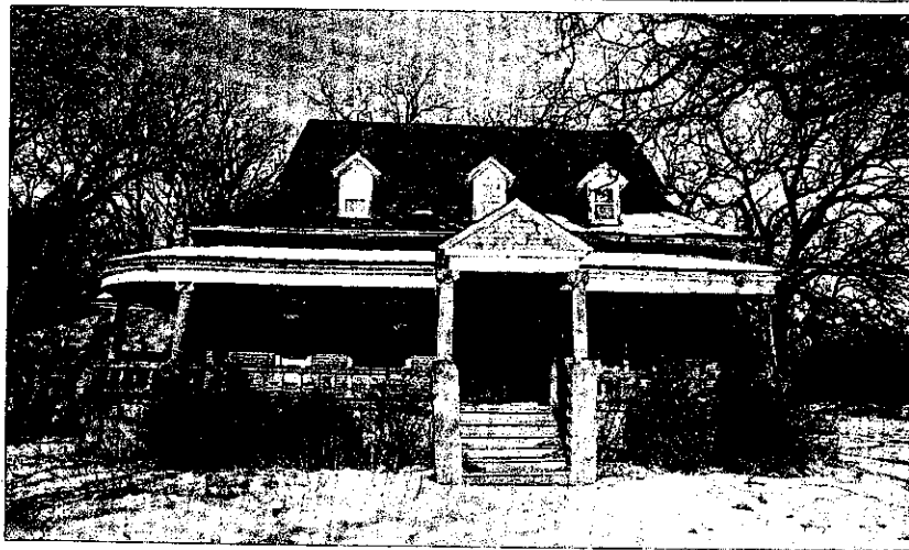
ON THE WAY OUT?: The future of the Lila farmhouse, E808 Plover Road, town of Plover, which was built around 1900, is uncertain due to the Highway 54 expansion project.
