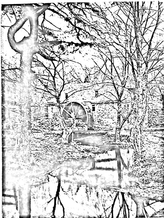
Robert's Mill, Church Lane and Wingohocking Creek
