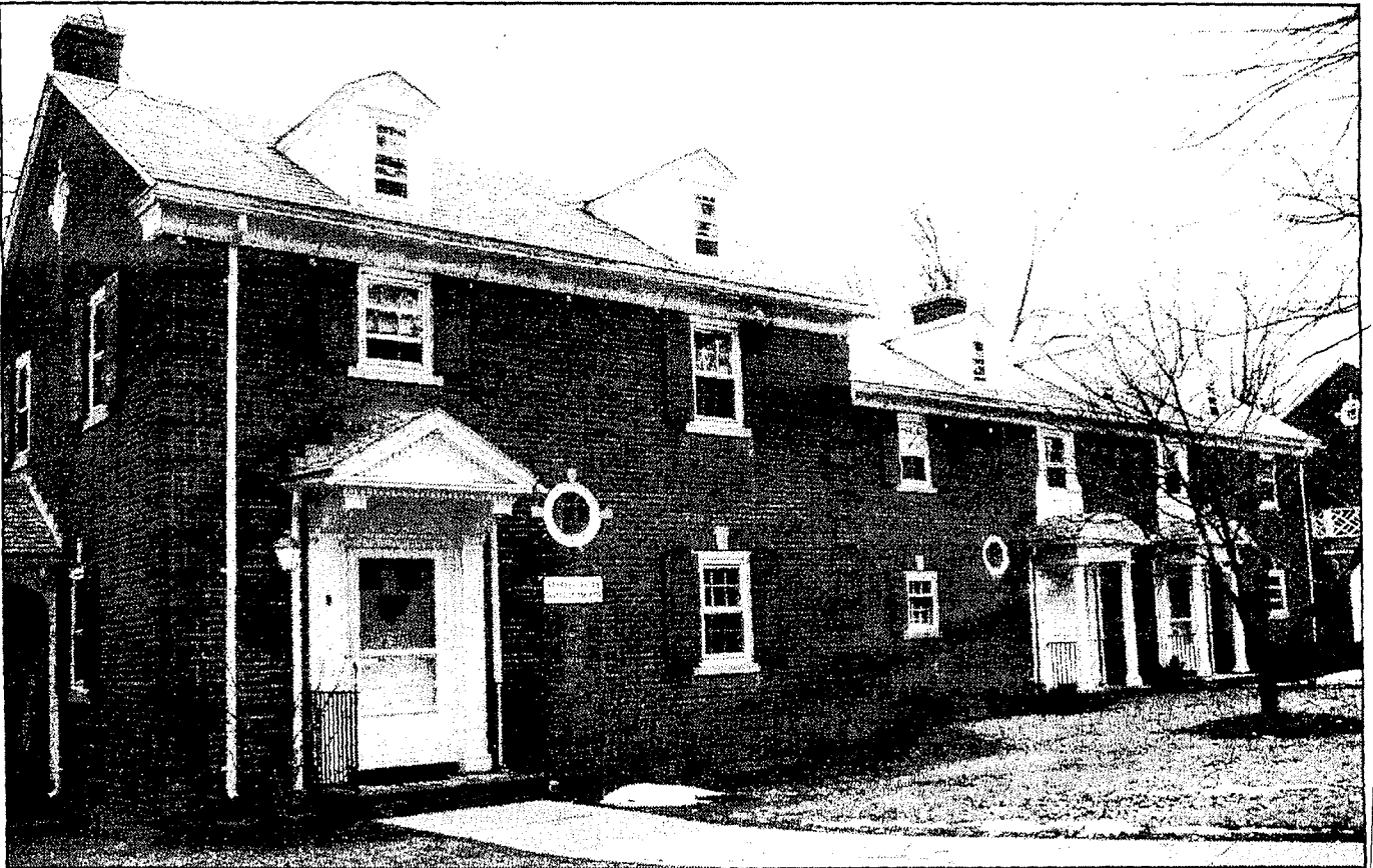
In the photo at top, GVCA information coordinator Salome Farraro stands in the middle of Apt. 3, which will be part of the New Deal Gallery. In photo at bottom, The buildings from left to right will be: a local and regional artist gallery, the New Deal Gallery and the GVCA offices. Space on the top floors will be used for art and music lessons.
