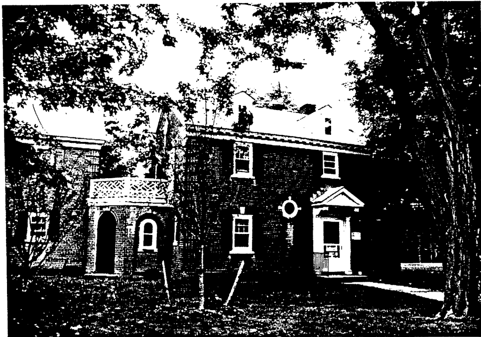
16) Building #4, east end, south elevation.
