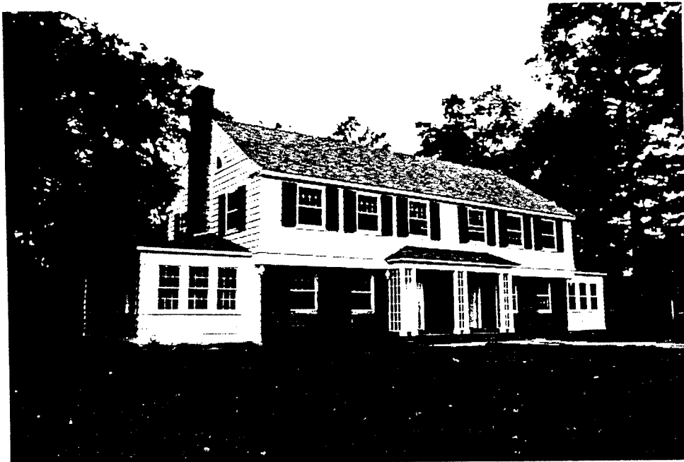
18) Double House (east of Building #6), west and south elevations.
