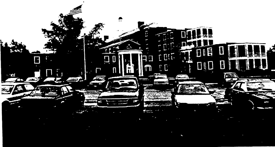
6) Building #1, west and north elevations.
