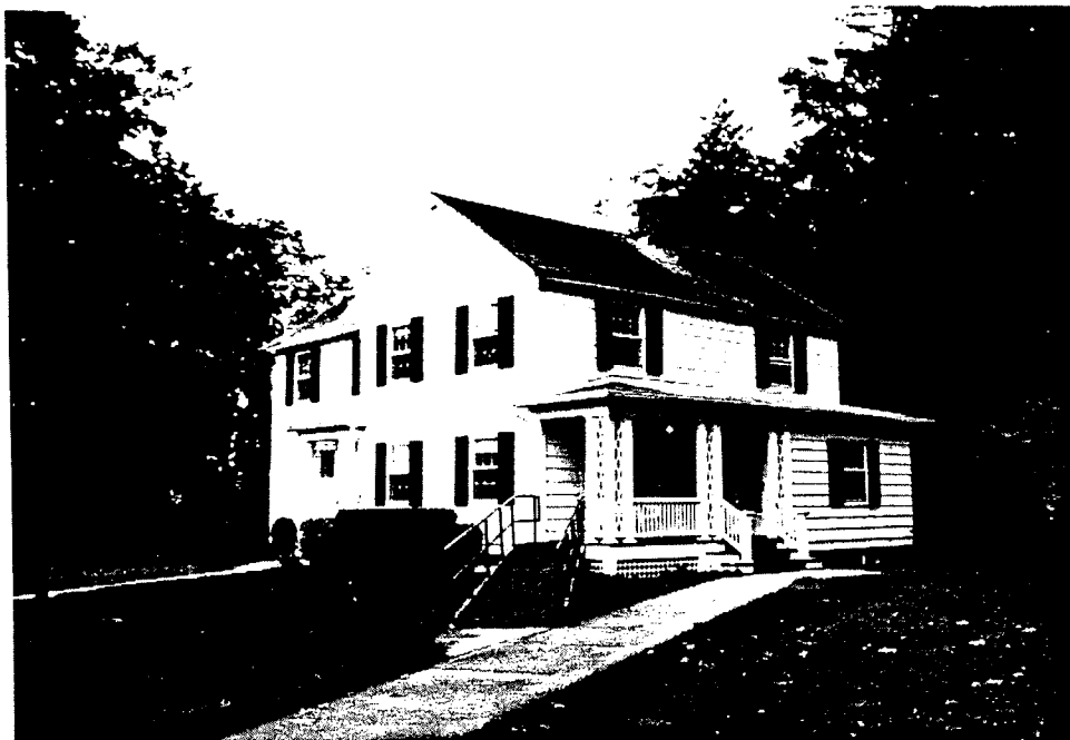
22) Building #8, west and south elevations.
