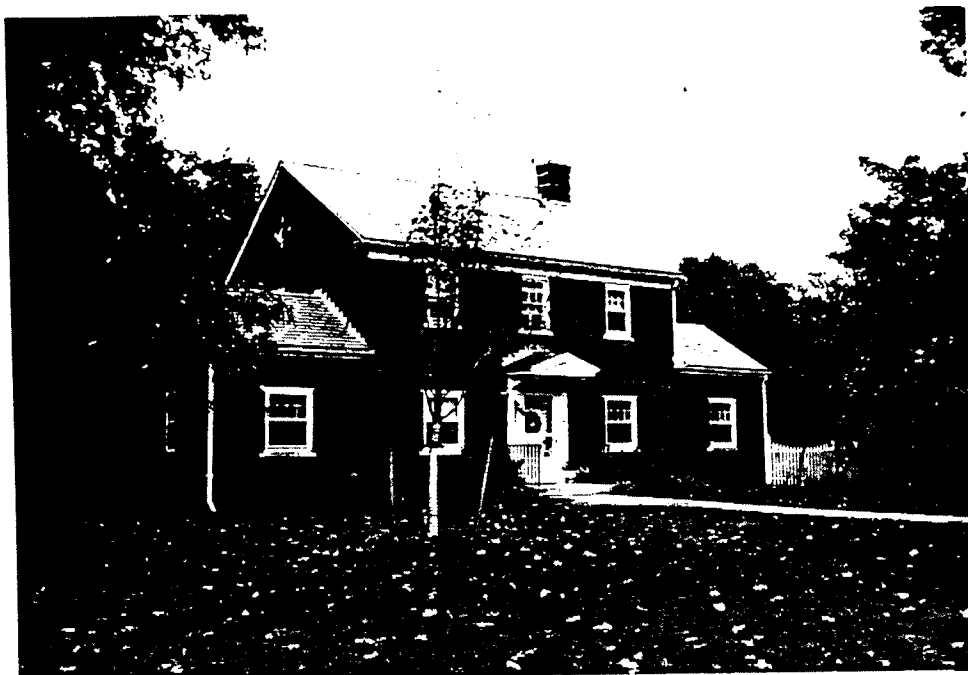
17) Building #5, west and south elevations.
