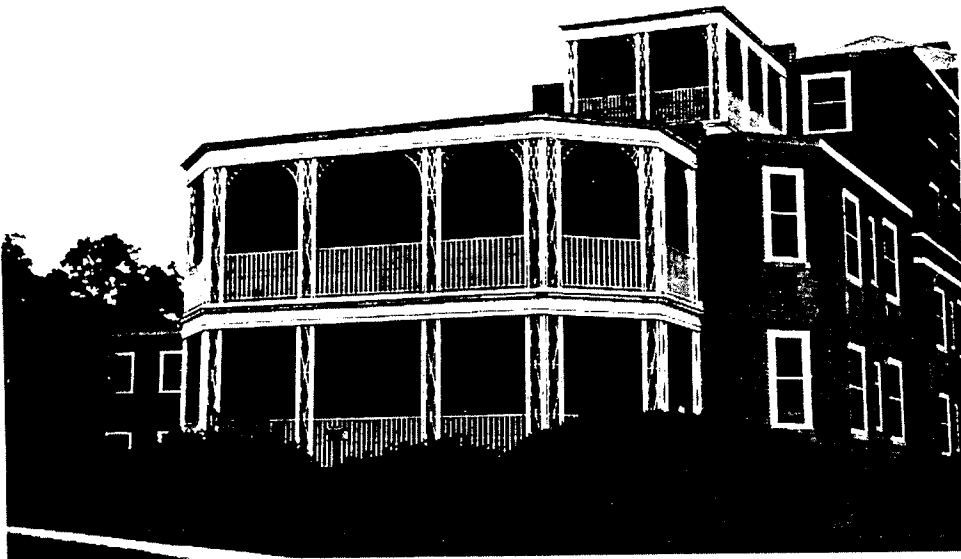
5) Building #1, west end porches at west elevation.
