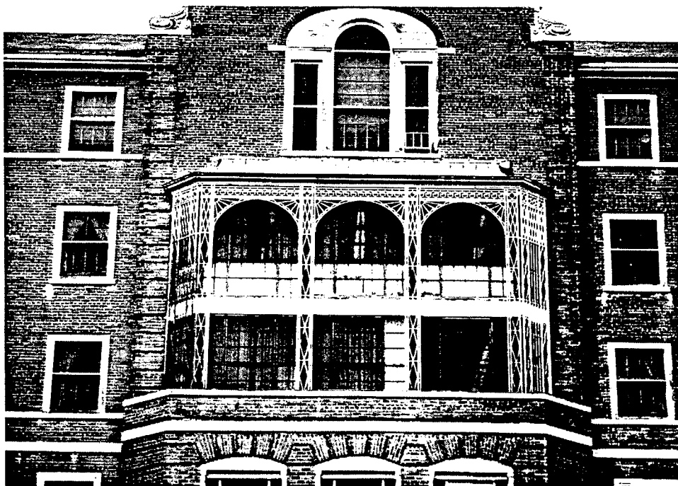
4) Building #1, central porch at south elevation.
