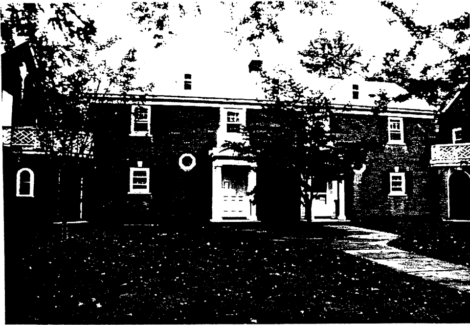
15) Building #4, center section, south elevation.
