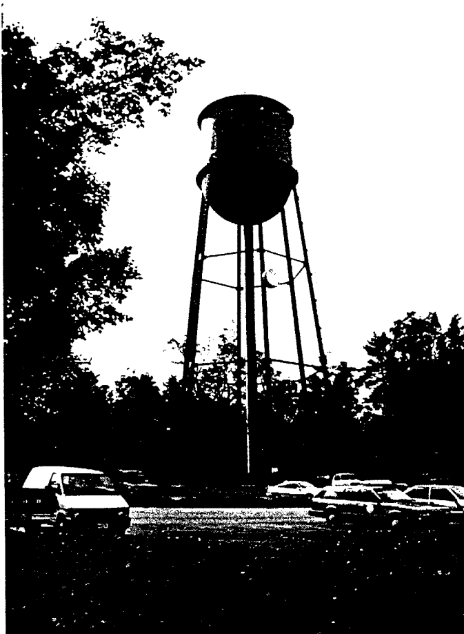
24) Water tower (south of Building #6).
