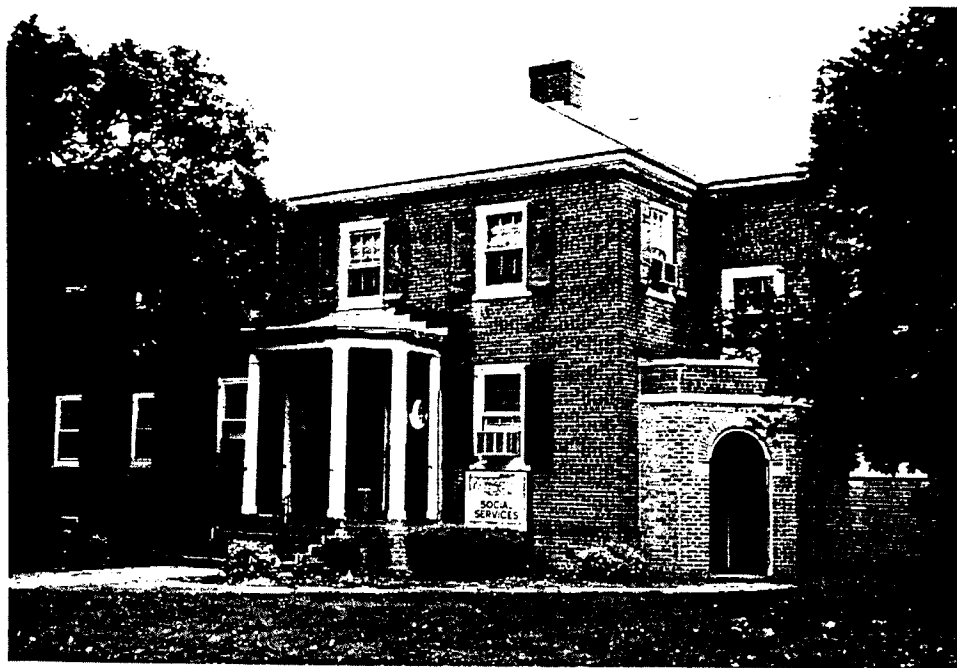
12) Building #3, central pavilion, west and south elevations.
