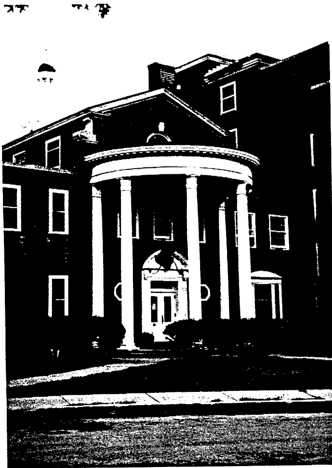
7) Building #1, curved portico at west elevation of northwest wing.
