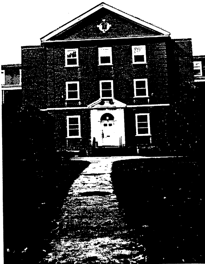
27) Building #2, central pavilion at south elevation.
