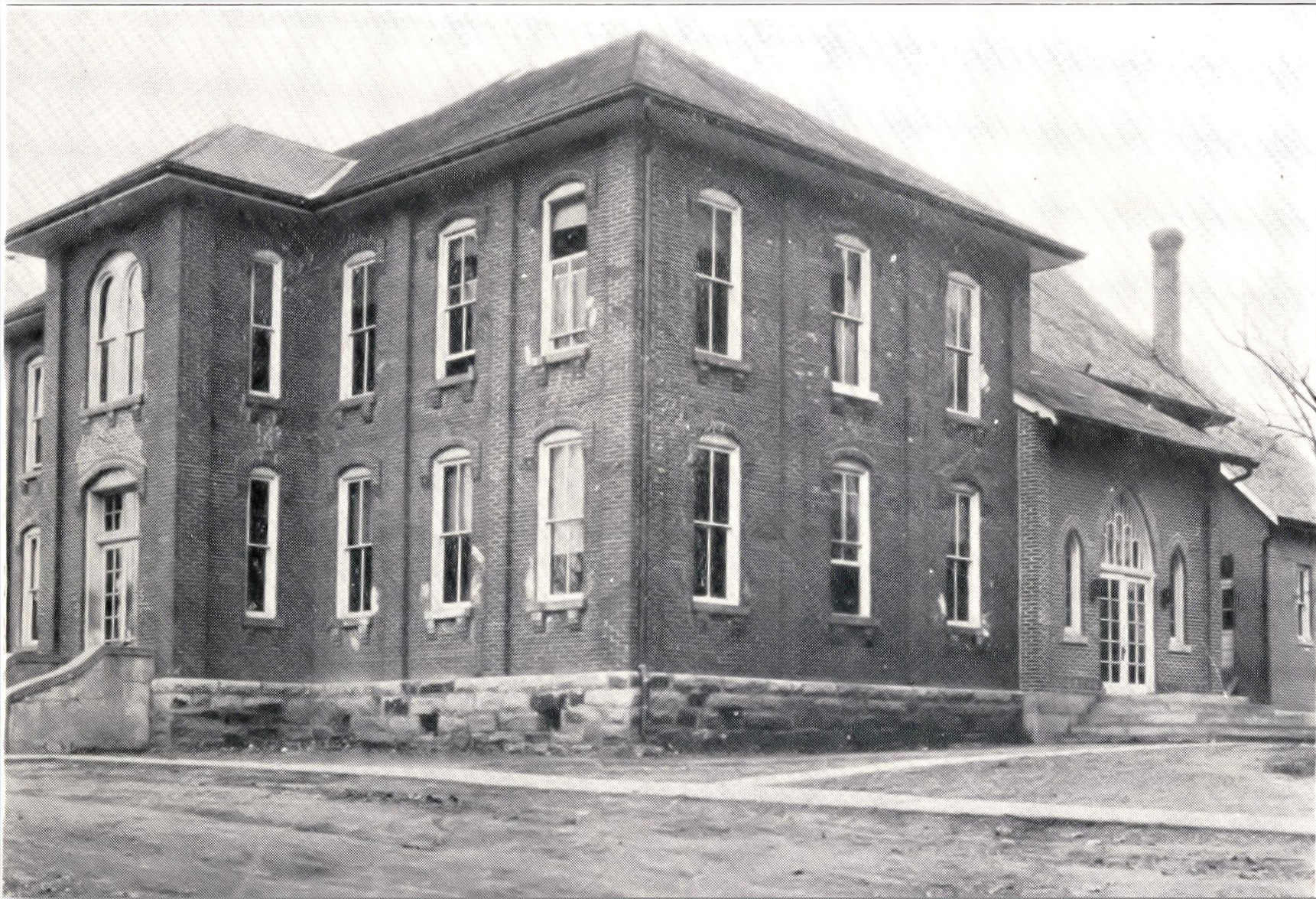
Mayfield Hall, 1920s, viewed from the southeast
