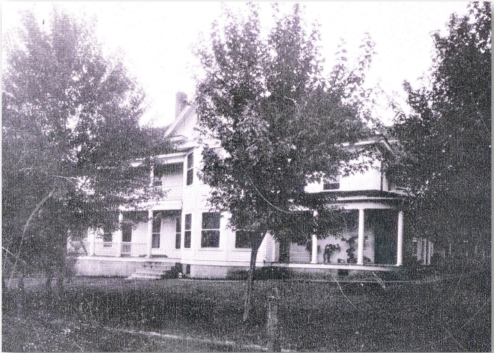
The Barton Snider house on High Street was acquired and renamed Franklin Hall. It was the men's dormitory.
