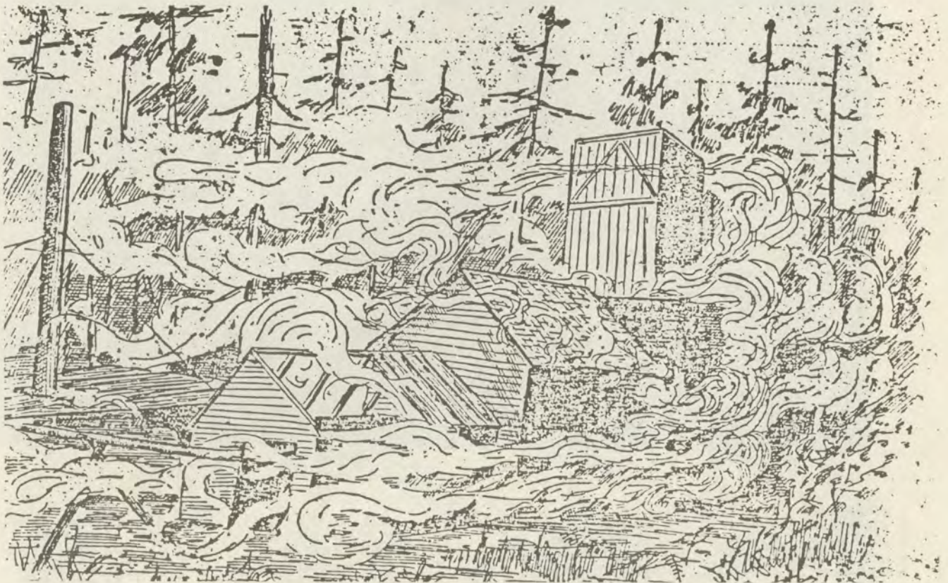
FAN HOUSE ON HILL SHOWING THE SMOKE FORCED ITSELF OUT AFTER THE OUTLET WAS CLOSED UP
