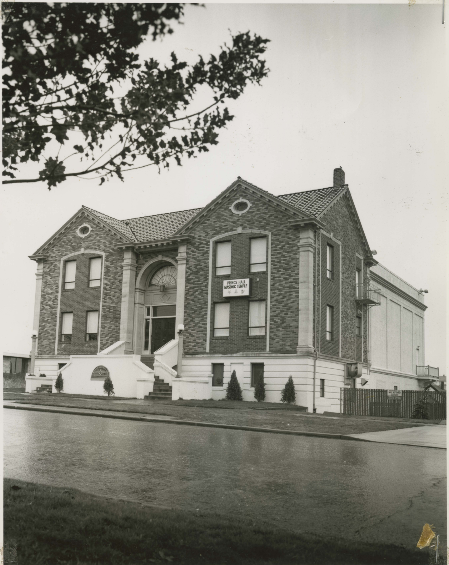
Present MASONIC HALL 306 24th St.
