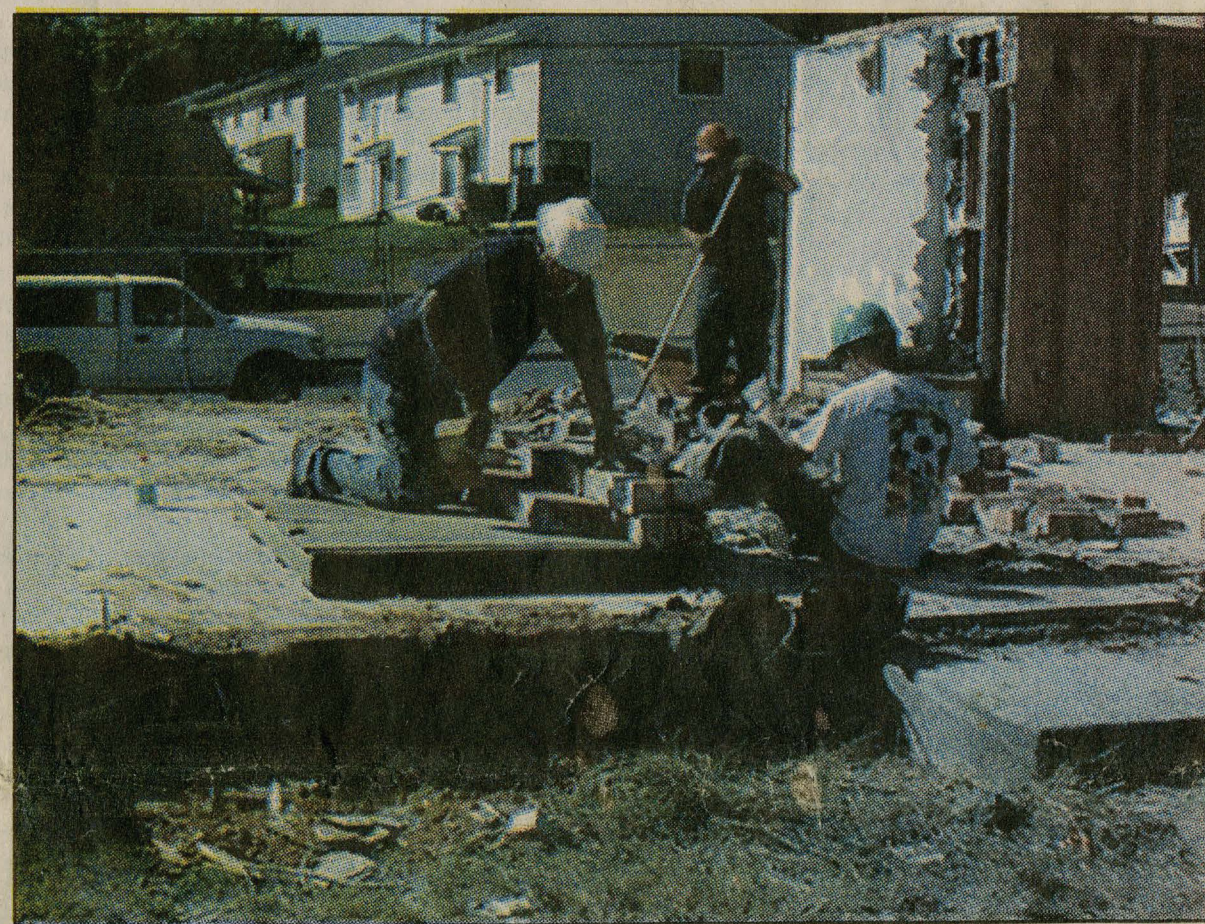
Crew members of Knight Construction take apart buildings at the High Point Housing Projects in West Seattle, and salvage vital parts. Photo/Shrinda Mitchell.
