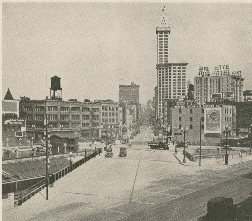
Lower Second Avenue, Repaved with Portland Cement- Concrete
