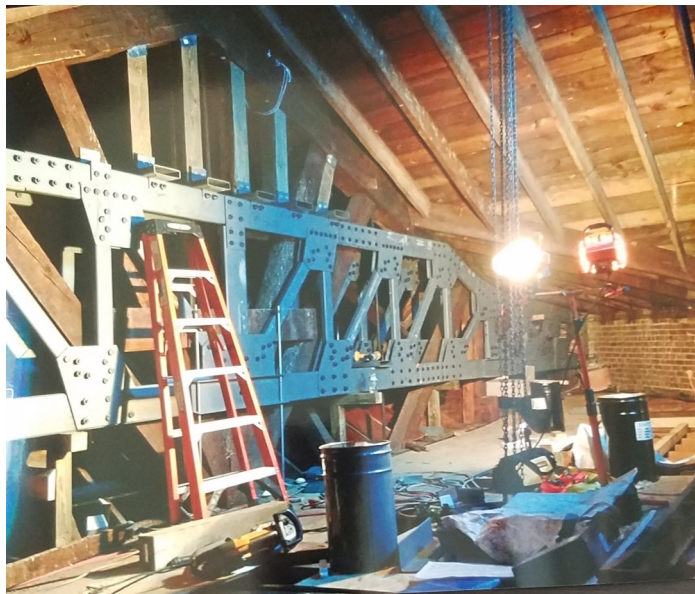
Steel reinforcements have helped stabilize the roof of the original Trinity Lutheran Church. (Photo courtesy of Rev. Toni Pate.)
