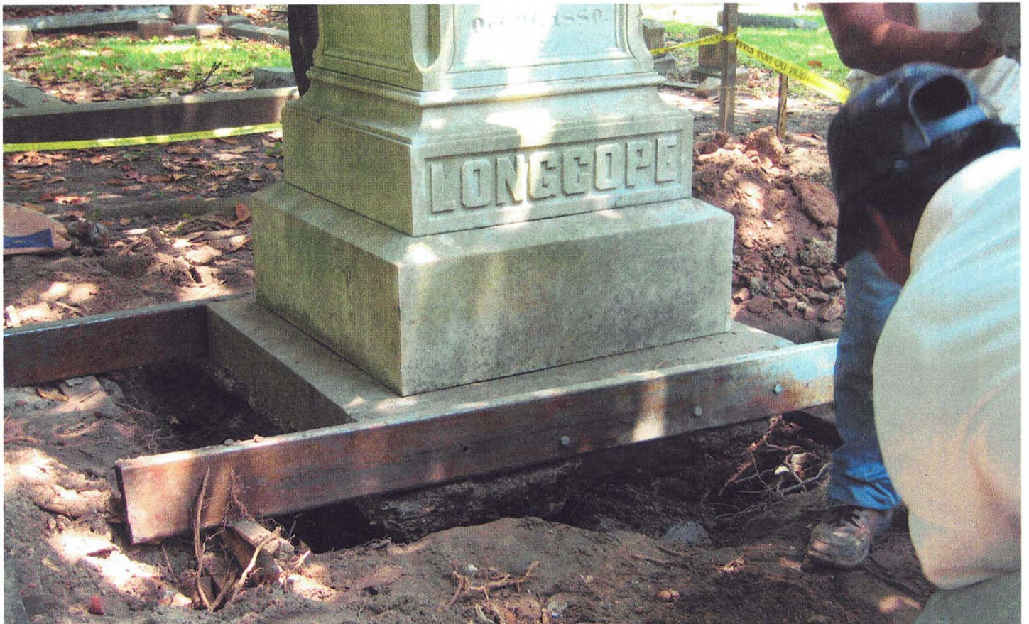
During restoration, the base was jacked up and leveled on a new foundation.
