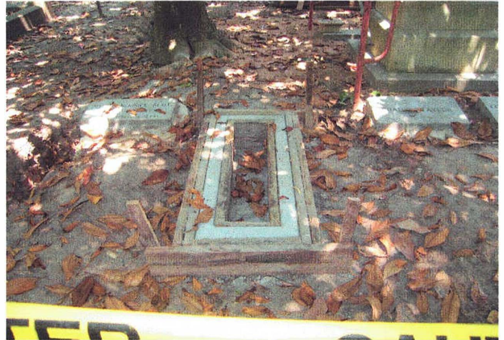
DURING: Small cradle in northwest corner of lot has been replaced; forms are still in place.
