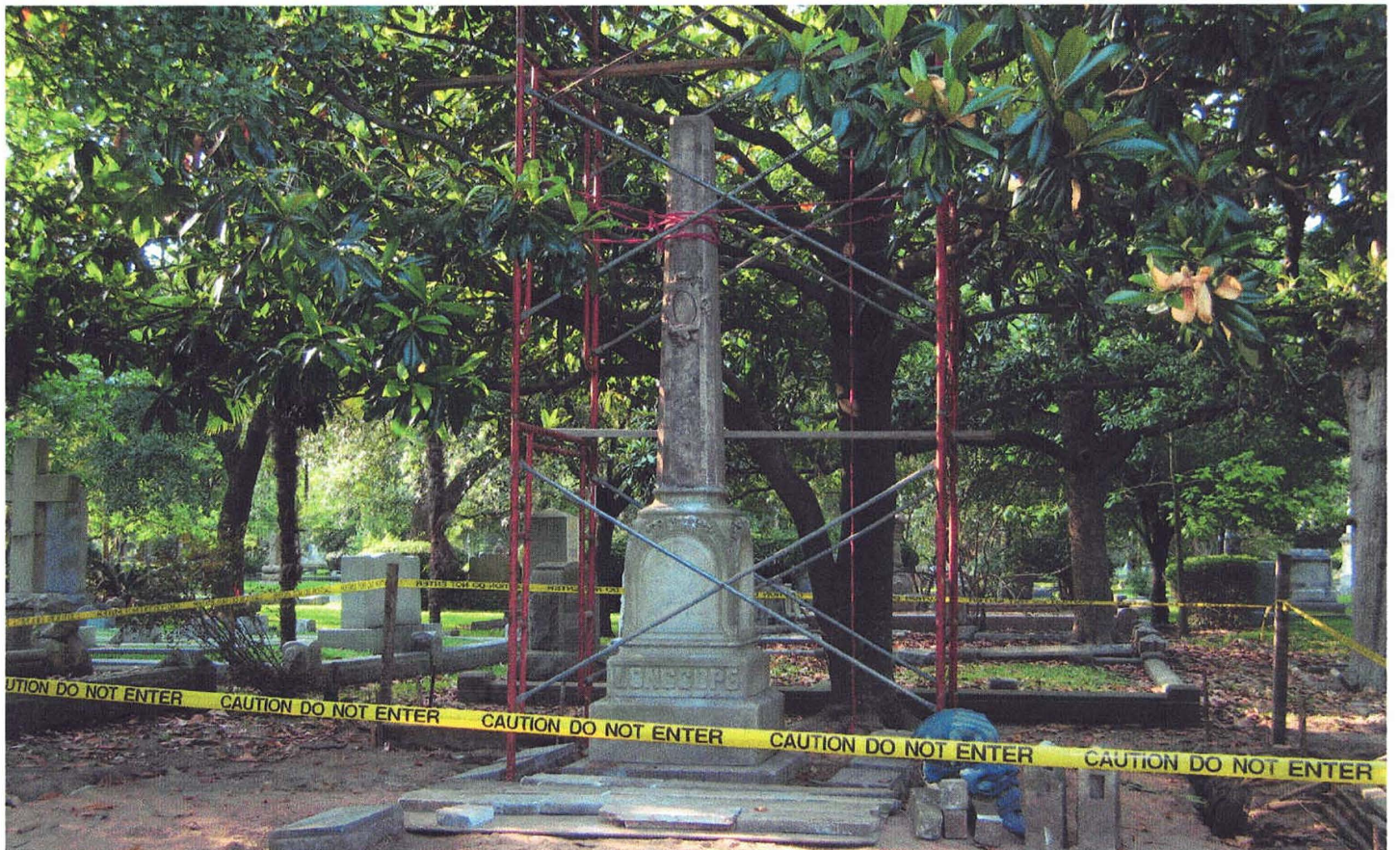
During restoration, scaffolding and a hoist were used to reset the shaft on the base.
