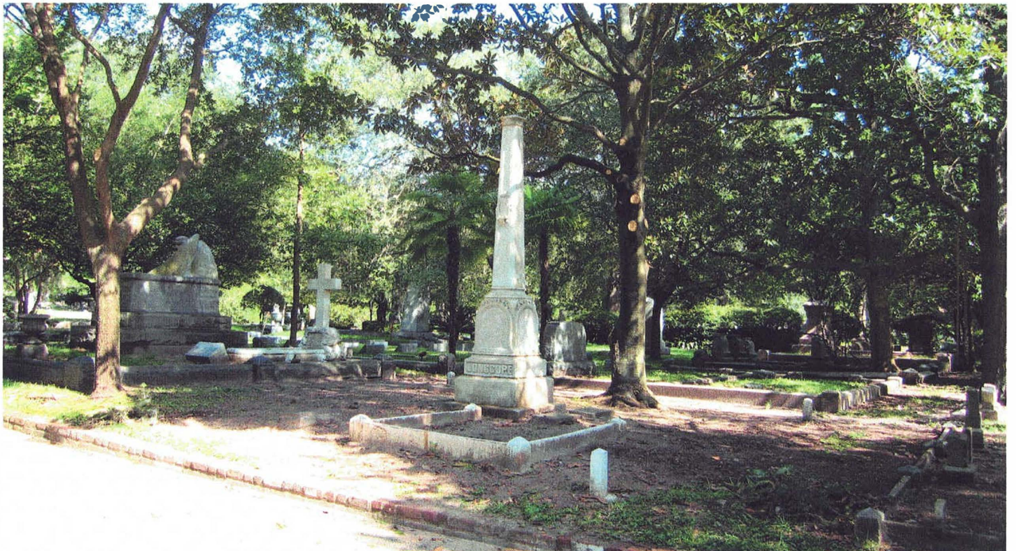
During restoration, the damaged coping was removed and the remaining marble corner posts were reset.
