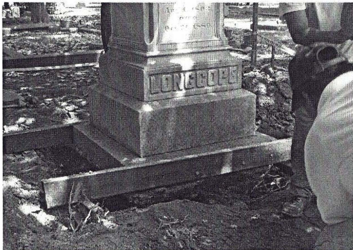
DURING: Steel beams are bolted to the base, which is suspended over an excavation for a new foundation. Remnants of the old cement and rubble foundation are still attached to the bottom of the base.
