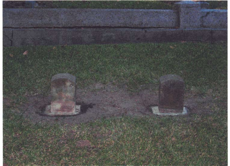
AFTER: The two small markers have been raised, leveled and reset on new foundations.
