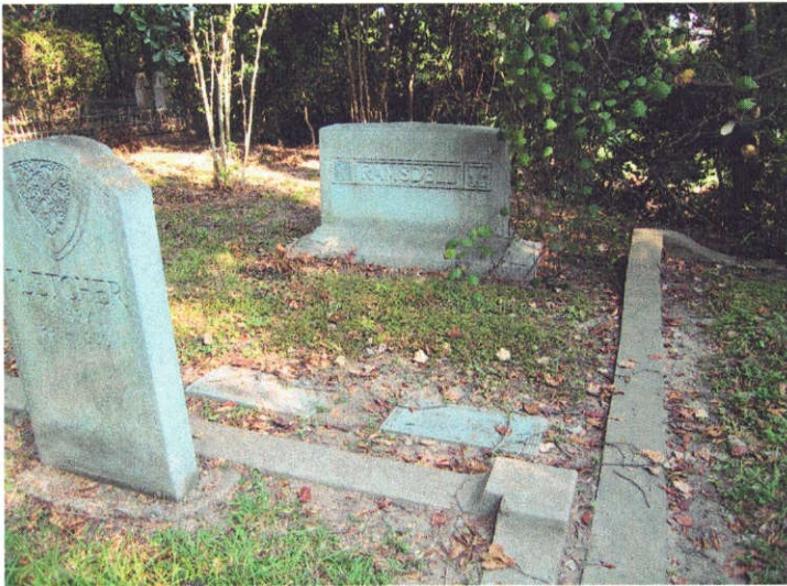
BEFORE: Two in-ground markers are sinking.
