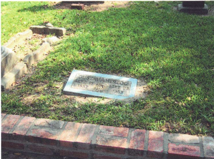
BEFORE: An in-ground granite marker had begun sinking.
