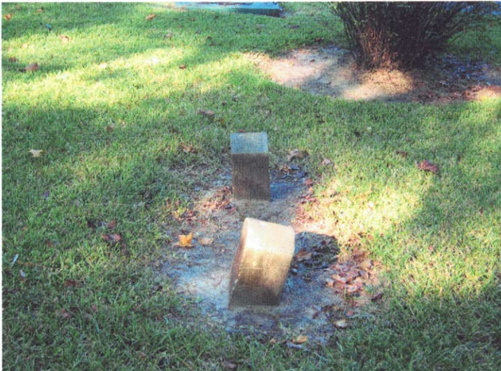
BEFORE: The two small marble markers are sunken and tilted.
