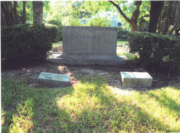
BEFORE: A raised, flat granite marker for Henry Bering was sinking 4° north.
