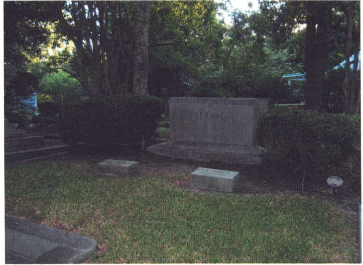
AFTER: The marker was raised level with the other marker on the lot and reset on a new foundation.
