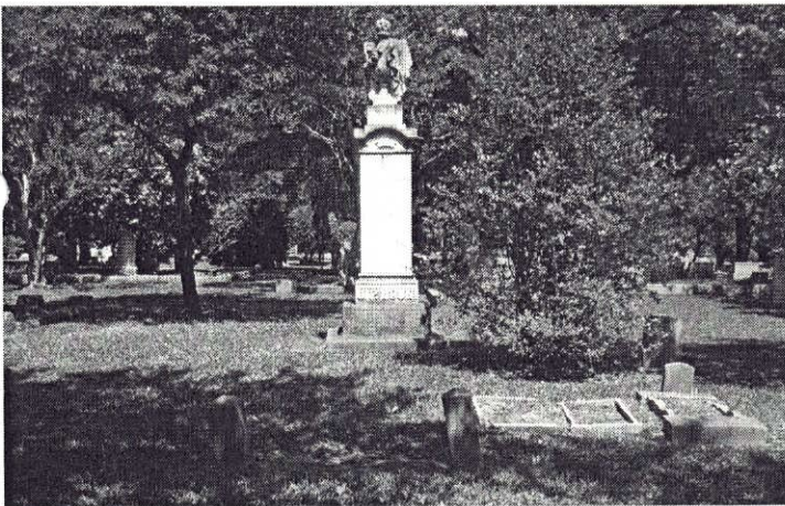
BEFORE: Restoring only the marble entrance would improve the appearance from the entrance road. The left entrance post is tilting 9\frac{1}{2}^{\circ} north and 2^{\circ} west, and the right post is tilting 10^{\circ} north and 2^{\circ} east.
