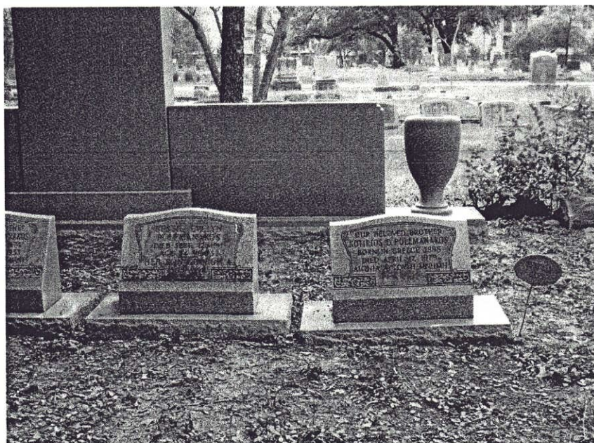
Before restoration - Marker for Sotirios Polemanakos is sinking
