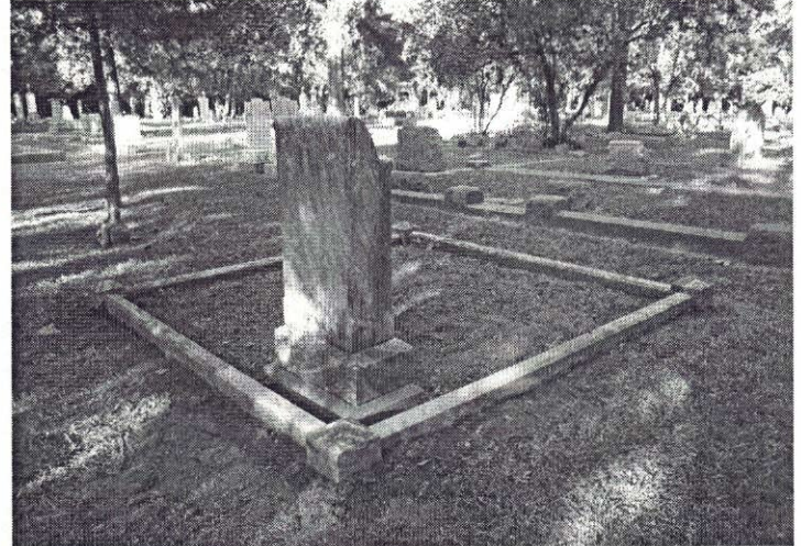
AFTER: The missing piece of the coping has been recovered and the four posts and the entire coping has been leveled and reset on a new foundation.
