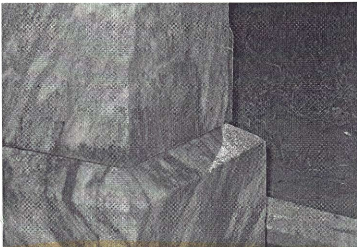
BEFORE: The monument is sliding on its base and overhanging the northwest corner approximately 1".
