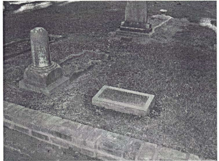
AFTER: The marker has been raised, leveled and reset on a new foundation
