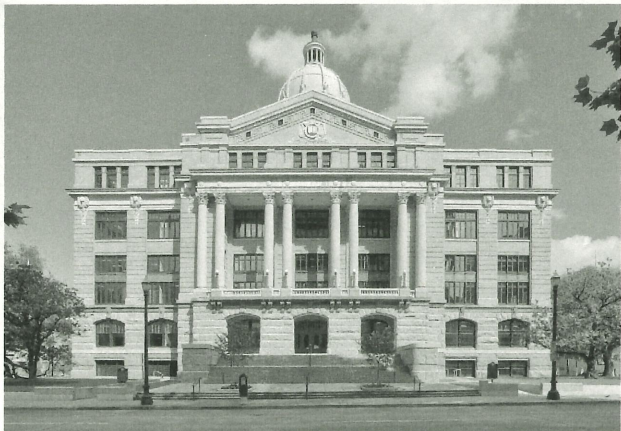
GHPA PRESIDENT'S AWARD HARRIS COUNTY Restoration of the Harris County Courthouse (1910) 301 Fannin Street Texas State Archaeological Landmark National Register of Historic Places Photo by Nash Baker Studios
