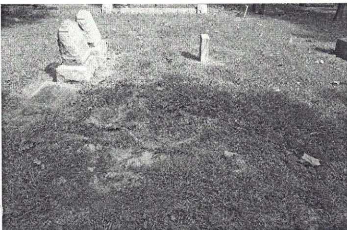
BEFORE: The ground surrounding an old tree stump on the adjacent 10'x10' to the east should be leveled and the sod replaced.
