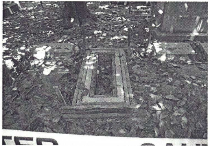
DURING: Small cradle in northwest corner of lot has been replaced; forms are still in place.
