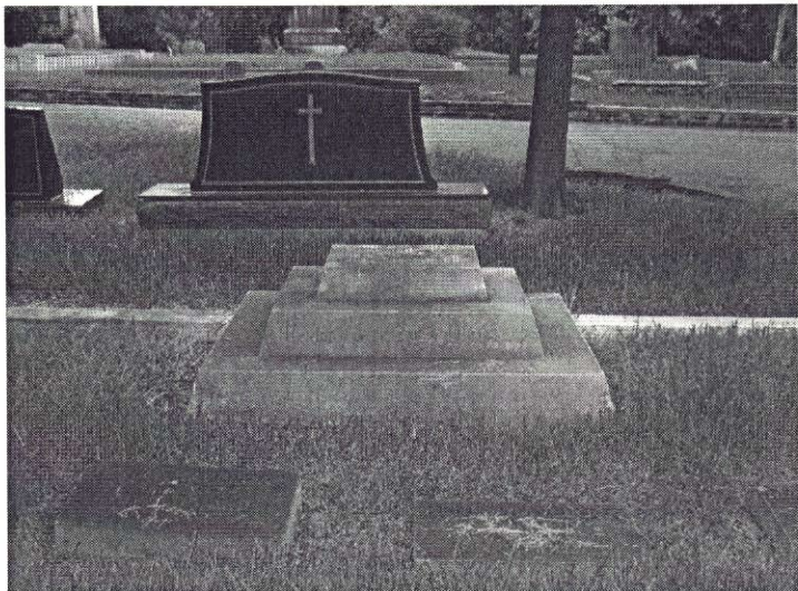
BEFORE: The base where the cross stood before being pushed over by vandals.
