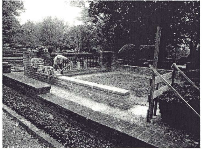
Leveling lot with top soil
