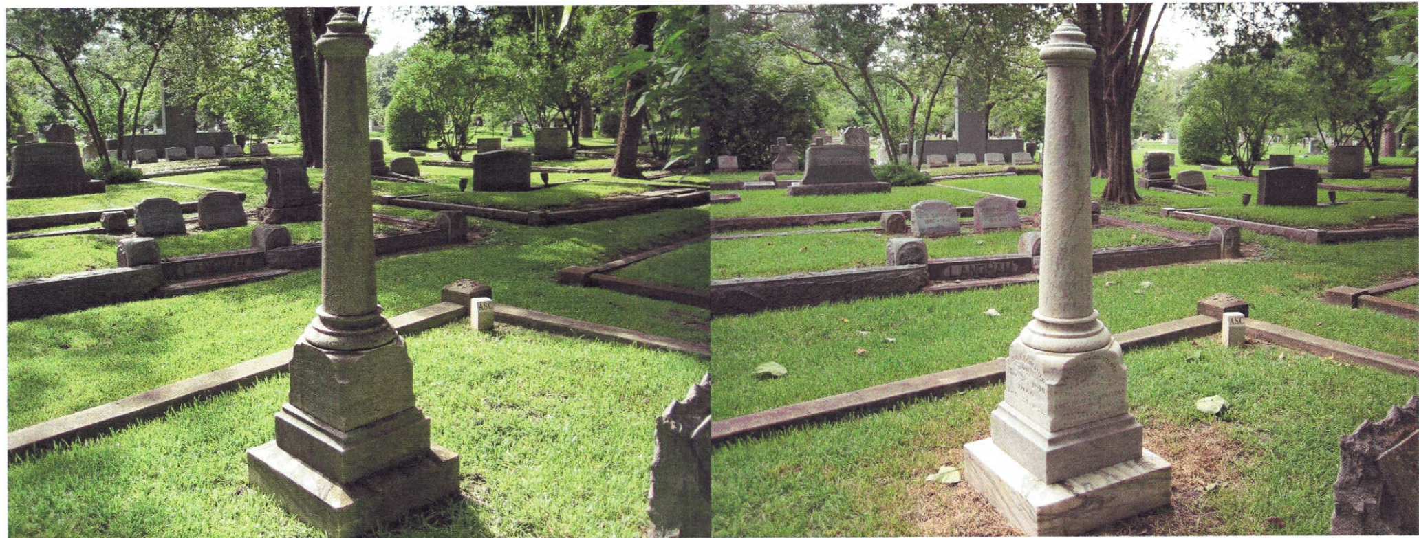
BEFORE: WA-260 Est. of M.J. Batchelder Finial Repair
