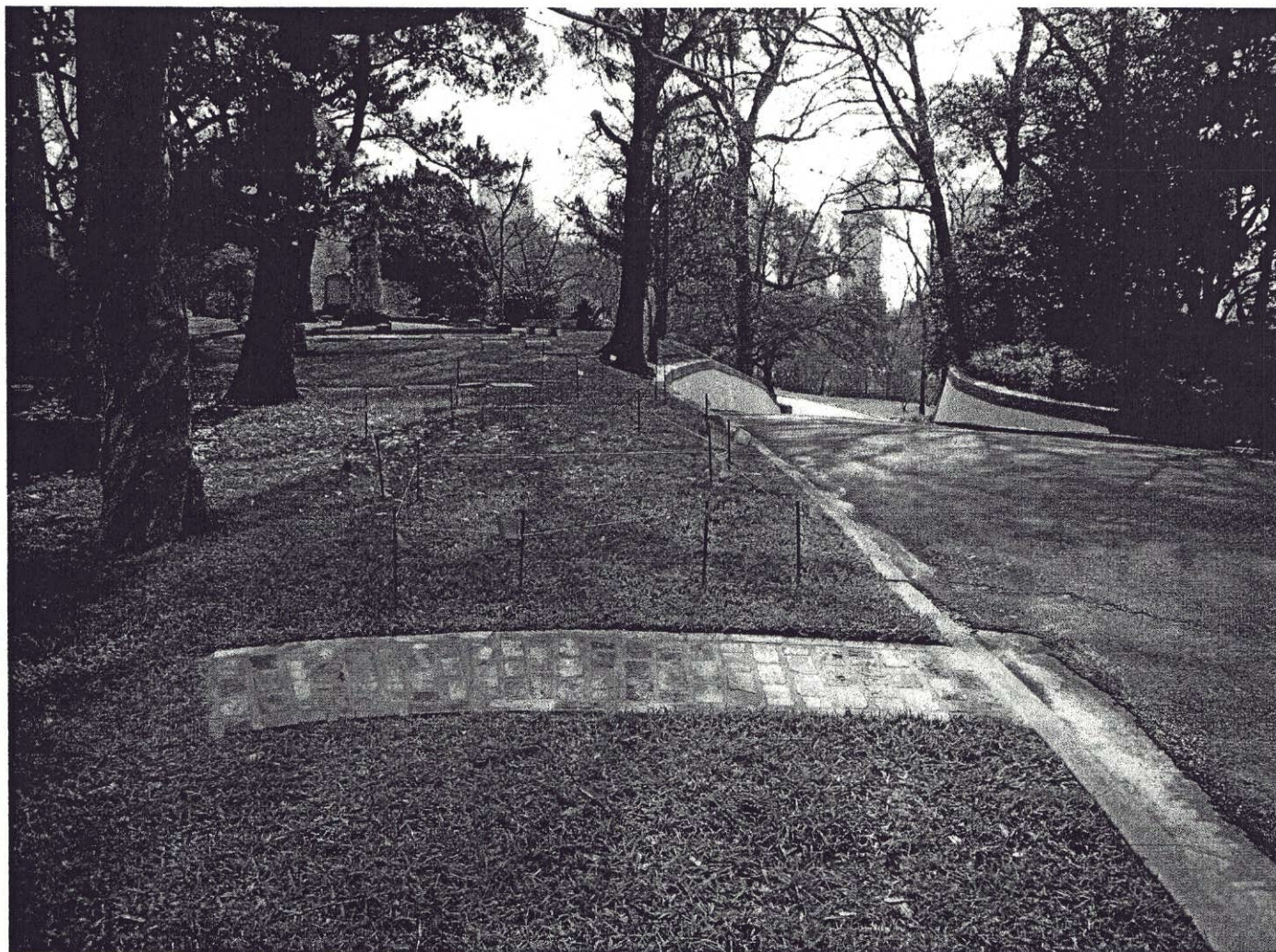
Construction of foundation and brick walkway
