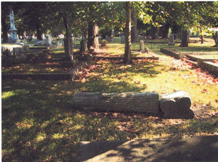
BEFORE: The base of the 6'-tall sandstone Woodmen of the World monument had tilted. The shaft had slid off the base.
