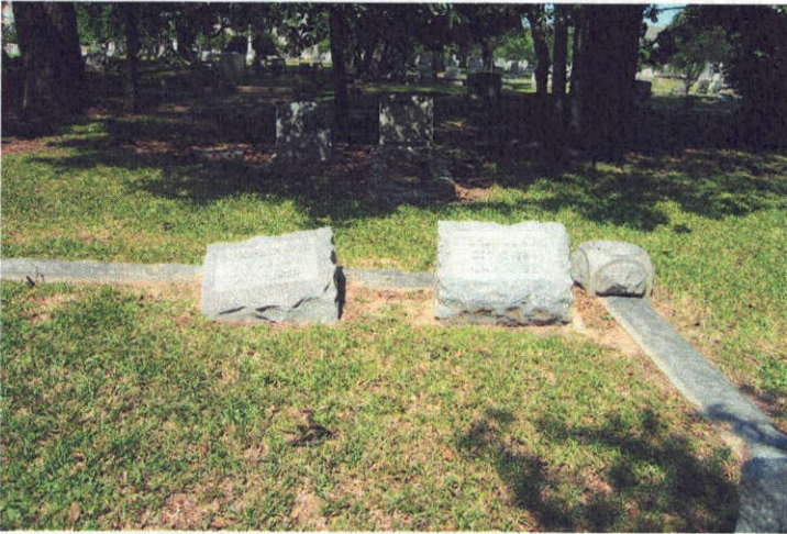
BEFORE: Granite headstone is tilting 11° south
