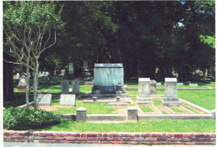
AFTER: The coping and entrance have been leveled and set on new foundations. Six marble cradles have been recovered, reassembled and set on new foundations. The small urns on the central tablets have been reset.
