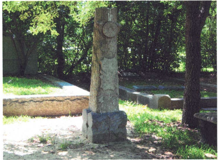
AFTER: The monument has been leveled and reset on a new foundation. The monument will be cleaned and the sod will be replaced.
