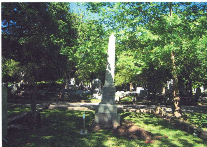
BEFORE: 10'-tall granite central monument is tilting 4° east.
