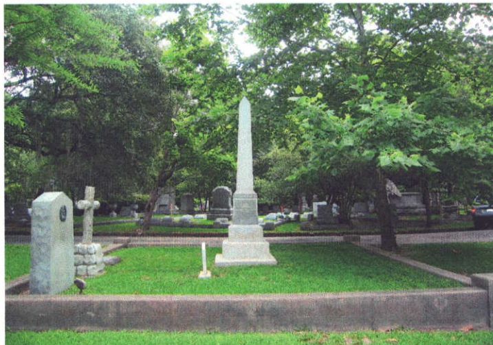
AFTER: The monument was reset on a new foundation and cleaned.
