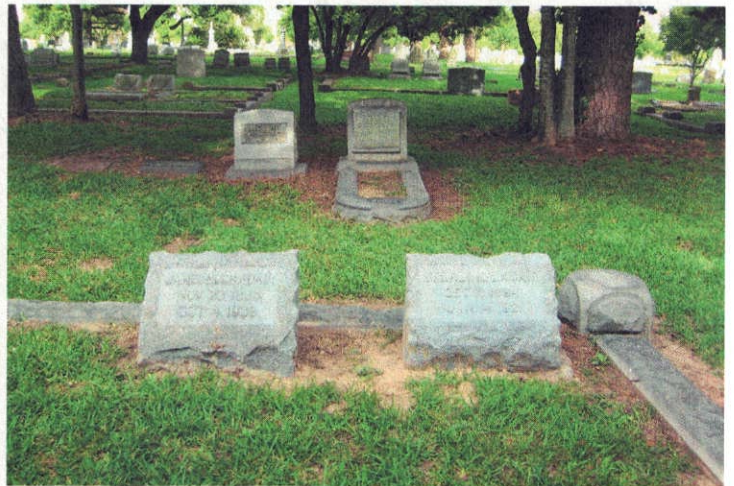
AFTER: Headstone has been leveled and reset on new foundation
