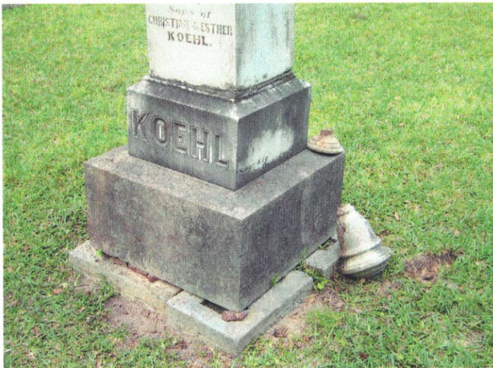
BEFORE: The monument is almost plumb, but has no foundation. It is sitting on concrete pavers, leveled by small stones used as shims. The broken finial is lying on the ground
