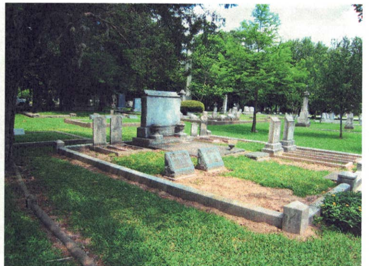
AFTER: All cradles on the lot have been reassembled, leveled and set on new foundations. The posts are plumb, and the coping has been reset on new foundations.
