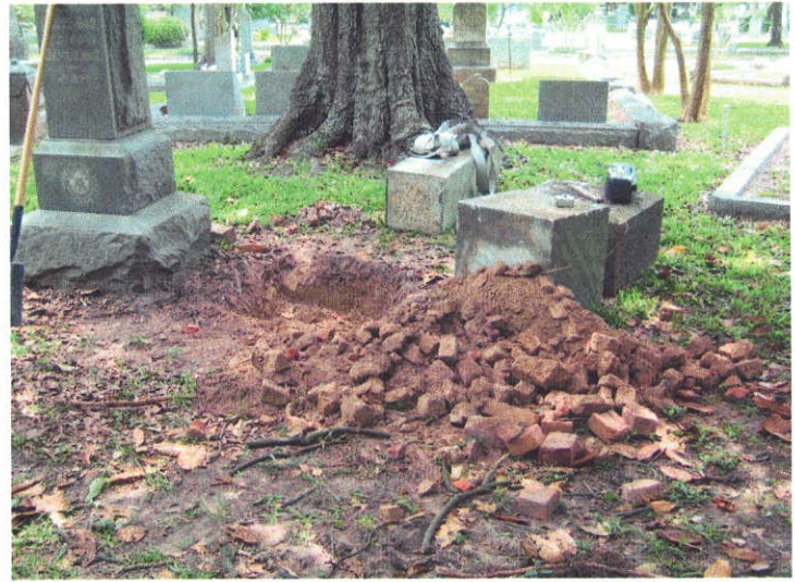
DURING: Excavation reveals only rubble for a foundation.
