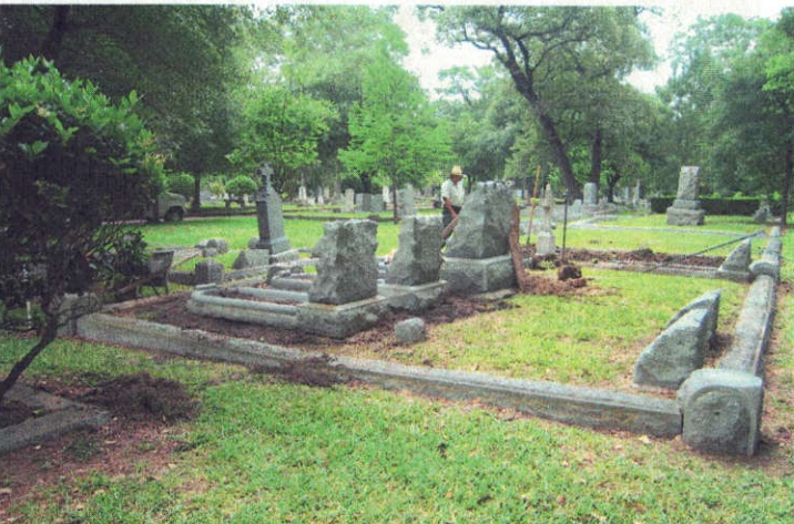
BEFORE: Coping on north and south boundaries is sunken toward the center. The photo above shows the north boundary.
