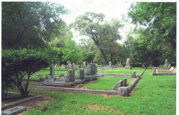
AFTER: Coping on north and south boundaries has been leveled and reset on new foundations. The photo above shows the north boundary.
