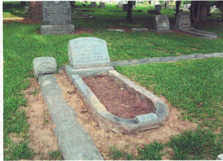
AFTER: The broken cradle has been reassembled, leveled and reset on a new foundation. The headstone has been properly leveled and reattached.
