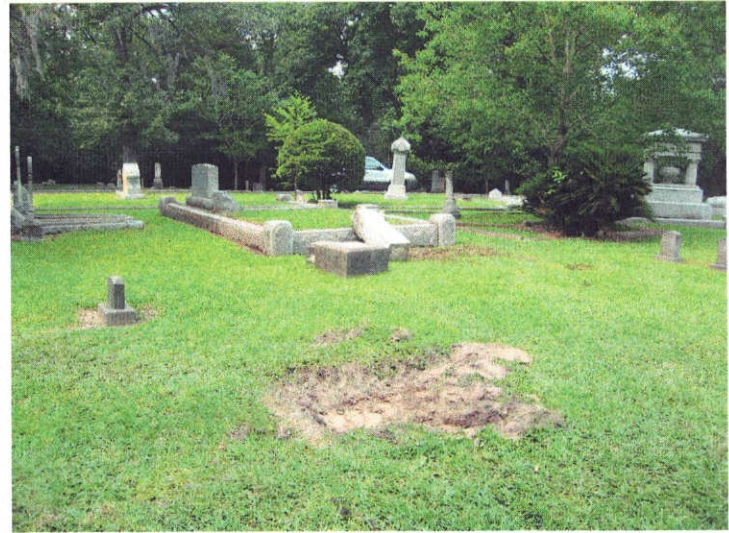
DURING: Excavation reveals no foundation under the 67"-tall monument.
