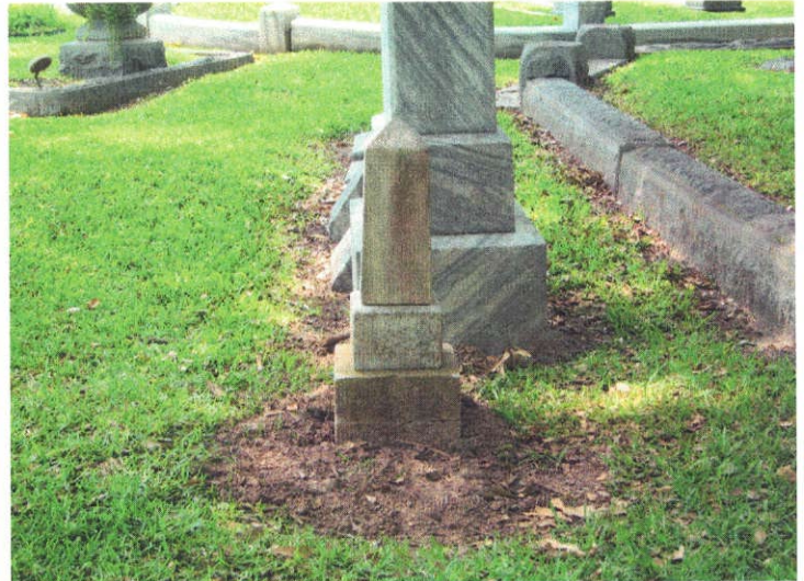
AFTER: The marker has been leveled and reset on a new foundation, and the upper portion has been secured to the base to prevent loss.
