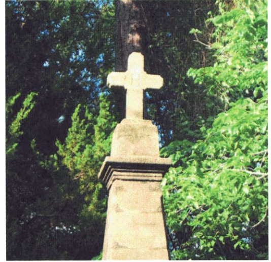
AFTER: The cross was repaired to prevent its being lost. Restoration of the entire lot and cleaning of the monument will be undertaken at a later date.
