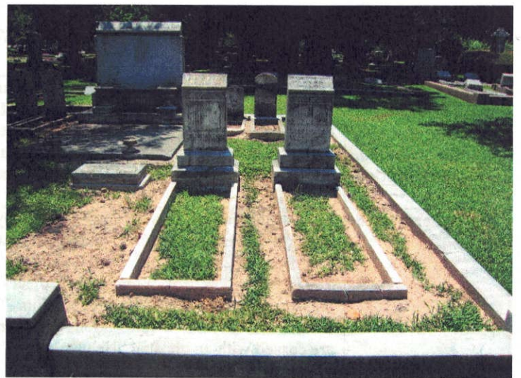
AFTER: All pieces of the cradles have been recovered, reassembled and reset on new foundations. The marker on the left has been leveled and set on a new foundation.
