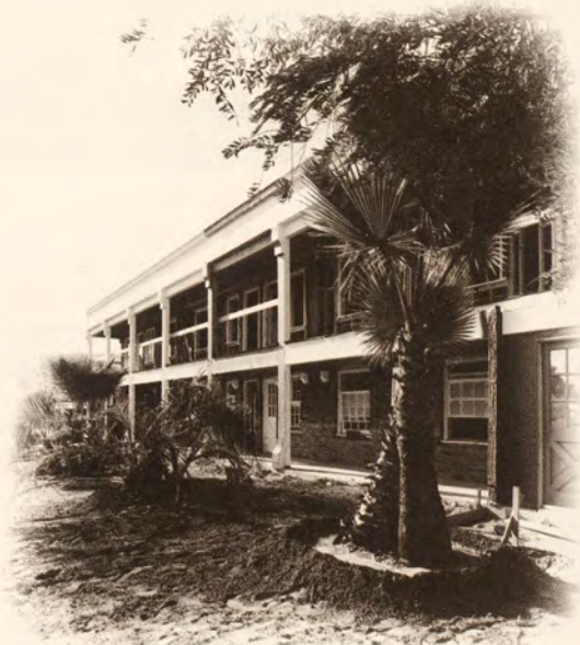
The old "Bandini" home today, completely restored.
