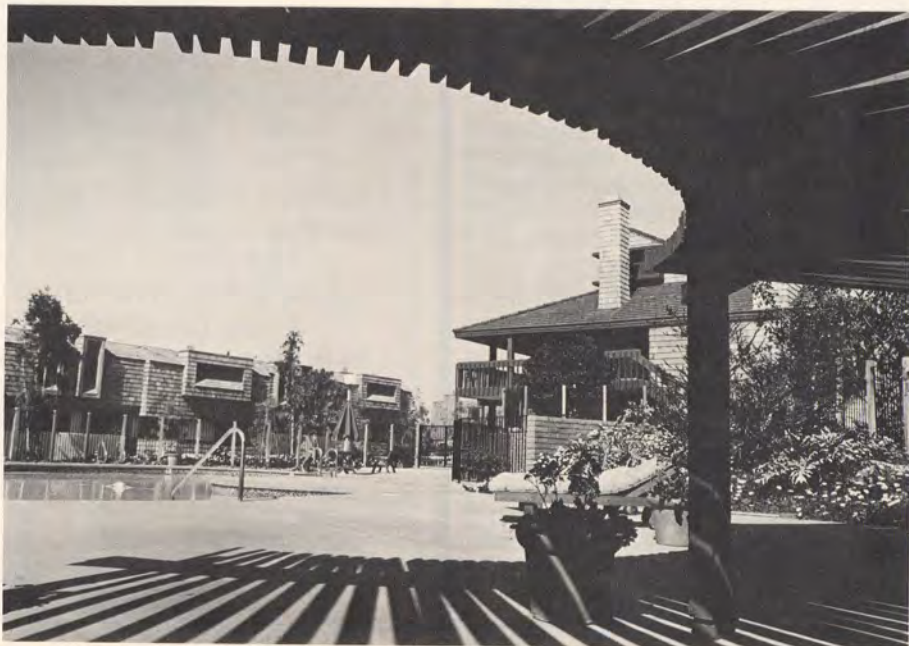
The lower recreational level of the richly appointed Sea Point Club (which includes a full-size kitchen) opens onto a wide lounging deck surrounding a large free-form swimming pool and whirlpool bath. Night lighted tennis courts are also a part of the recreational facilities at Sea Point Townhomes.
