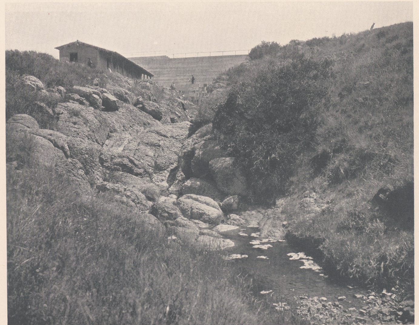
Nature made an alluring spot of this little ravine below the dam and pumphouse on the Fairbanks-Pickford estate. Yes, those are lilies in the pool.
