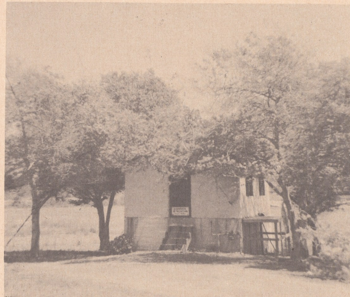
The old Sewage Treatment Building which served Rancho residents for over 25 years. This building will be razed in the near future.
