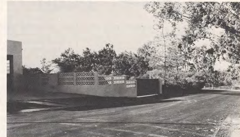
Santa Fe Irrigation District's new equipment and storage area
