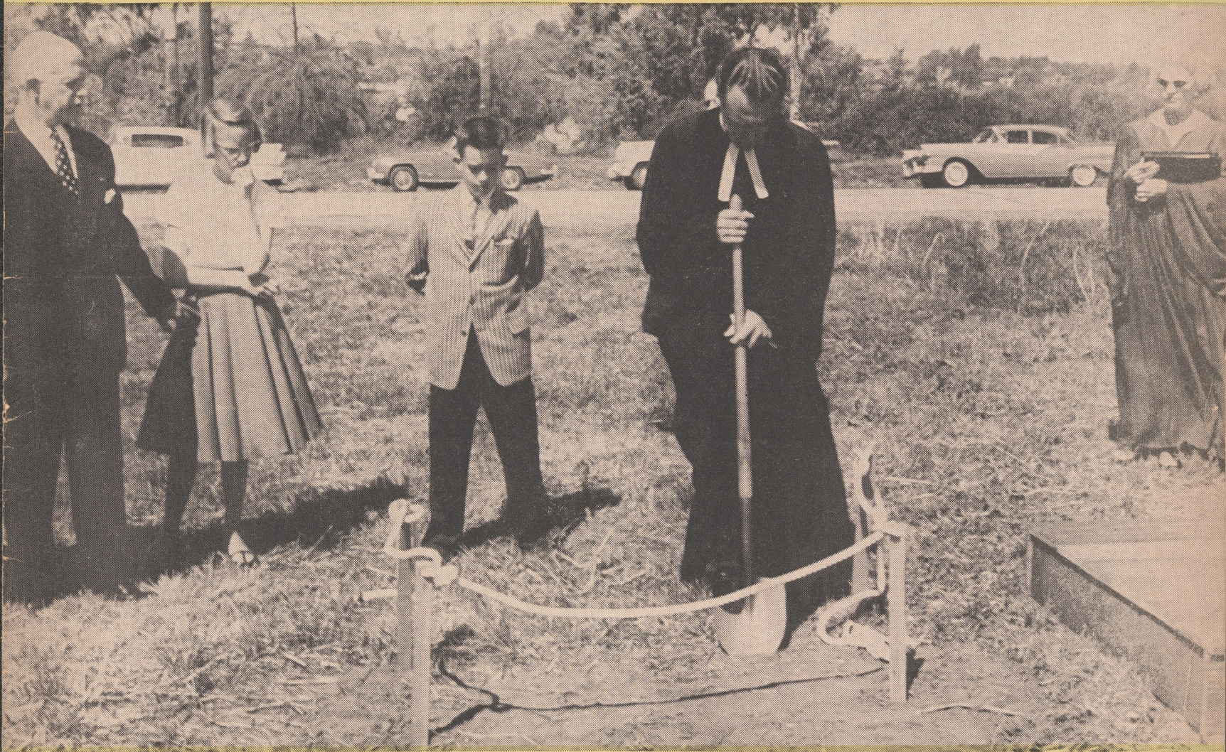
FIRST SHOVELFUL — Rev. Chester L. Tolson lifts the first shovelful of dirt in the groundbreaking ceremony for the new Village Church, held March 15. His son, Steve, stands back of him with Dr. Herbert Willy Meyer and Susan Kelly also looking on. Work is well started on the new building.
