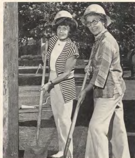
Grace Burns (left) and Edna Pulver, who have spearheaded the Patrons of Palomar College clock tower project for the past three years, are shown helping to erect the first of four 50-foot utility poles. Their hard hats, together with the poles and the job of erecting them, were donated by San Diego Gas and Electric Company. (Photo by Dale Oshima)
