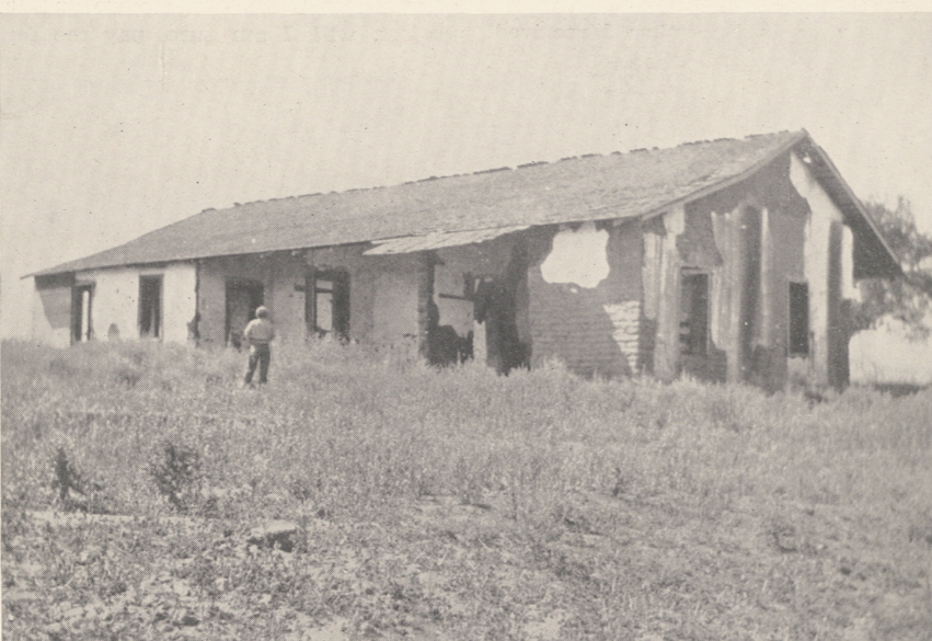
This is the way the old Osuna house looked before A. H. Barlow took it in hand. Notice adobe walls, 3 feet thick. Now see the reconstructed home on next page.
