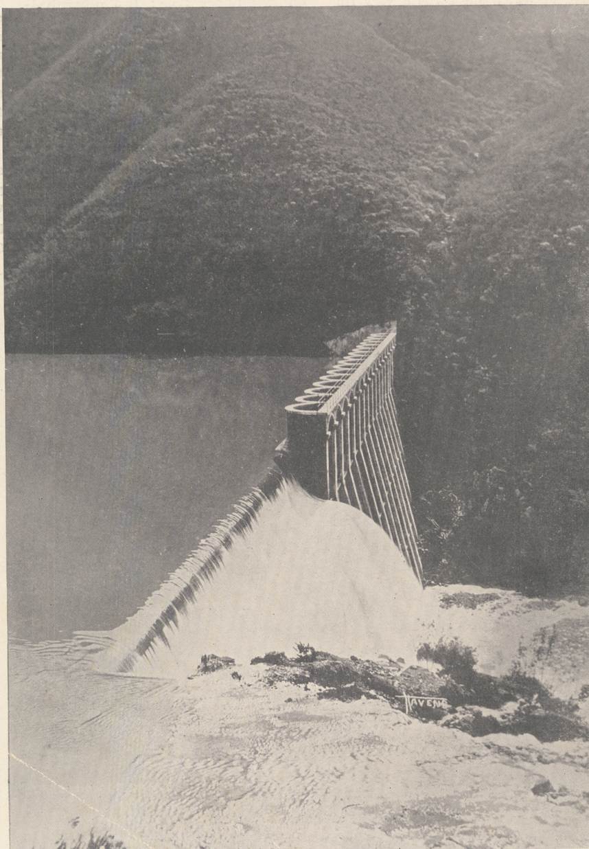
There is a definite feeling of power and ampleness in this early photograph of Hodges Dam, source of Rancho Santa Fe water
