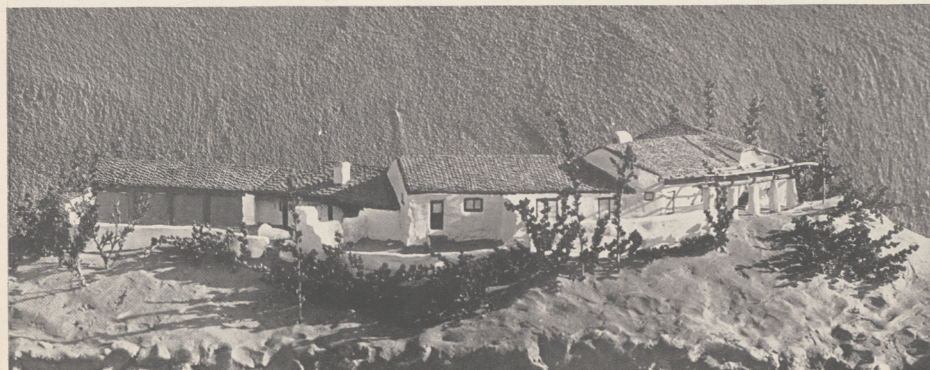
The Cord home as it will appear from the Olivenhain Valley side. Notice how cleverly the service court is cut off from the main terrace by high walls. Imagine the view Mr. and Mrs. Cord will have from this many-angled home,
