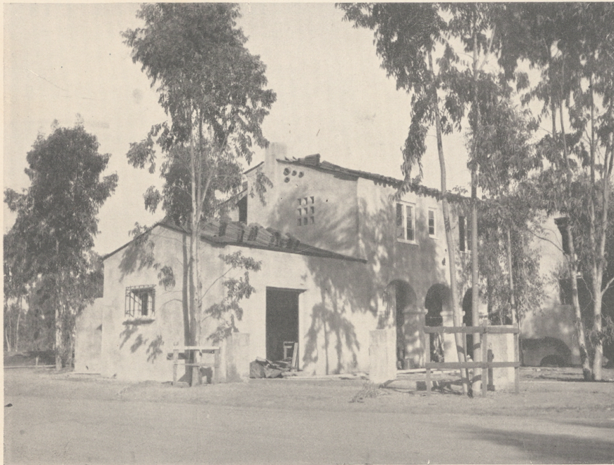
The Christiancy Apartments are nearing completion. They offer quite a contrast in architectural design to the boxlike apartment houses that ruin so many city streets.
