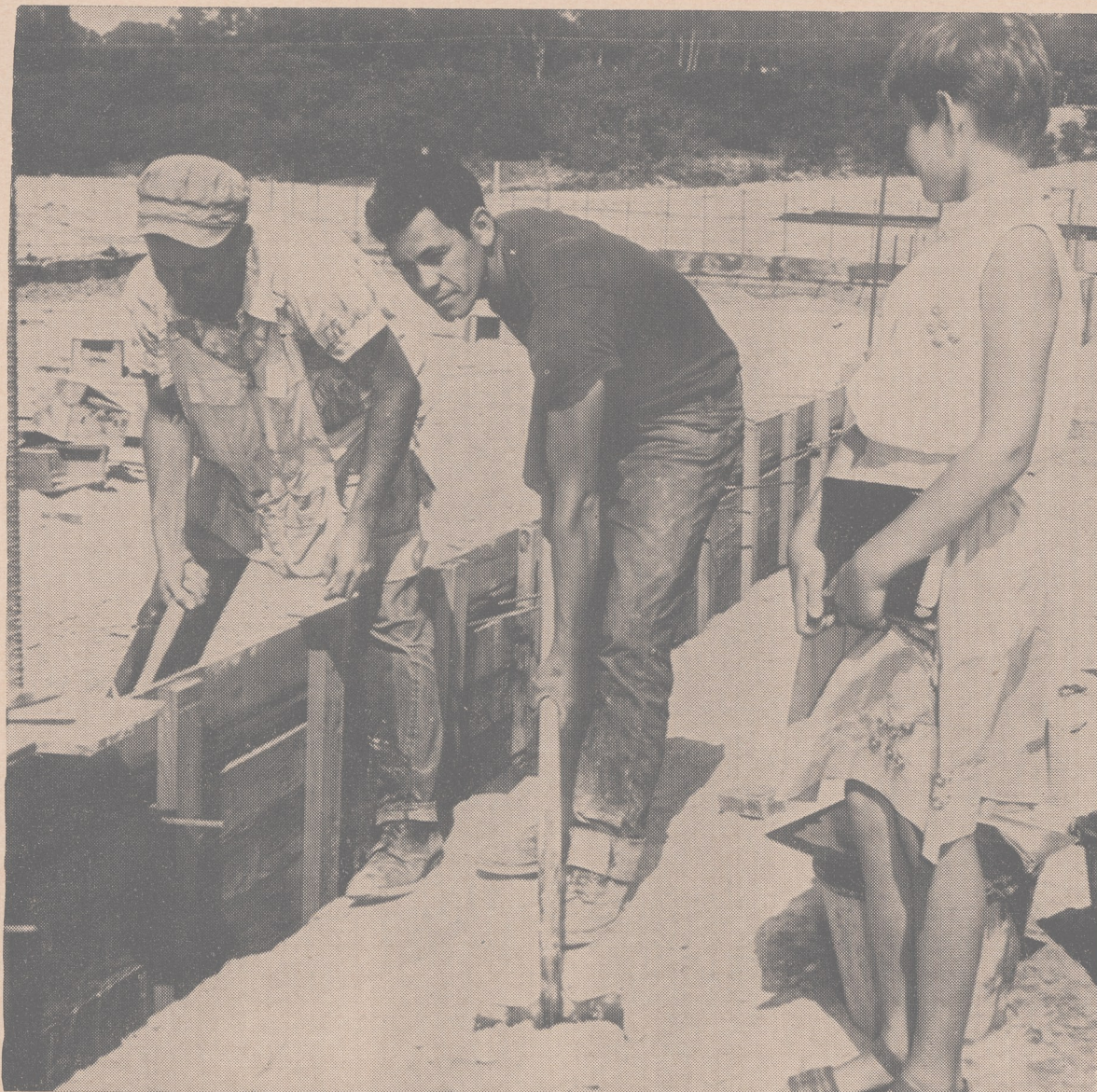
MARGARET ANN APERANCE, seven-year-old daughter of Mr. and Mrs. Bill Aeprance, went over to the site where the new Rancho Santa Fe Elementary School is being constructed to watch construction workers Bob Bedford and Robert Morones. The new school will be ready for occupancy October 15.
