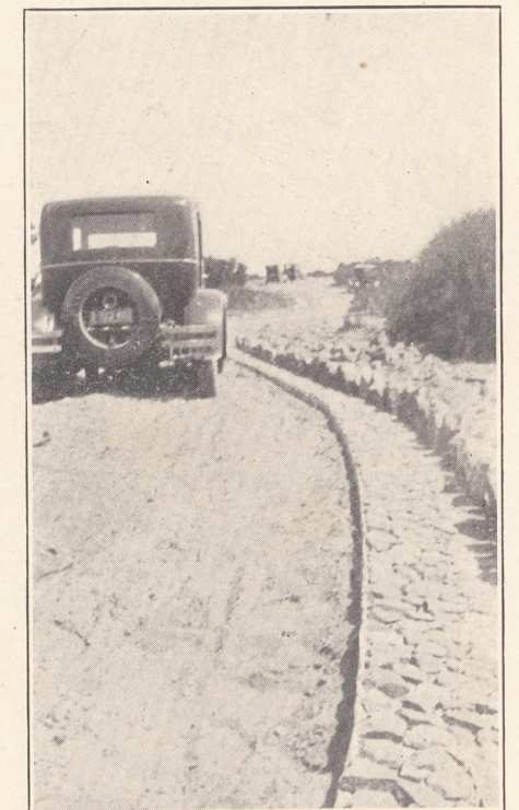
Grouted gutters and curbs of native stone are unique features of Mr. Keck's development.
