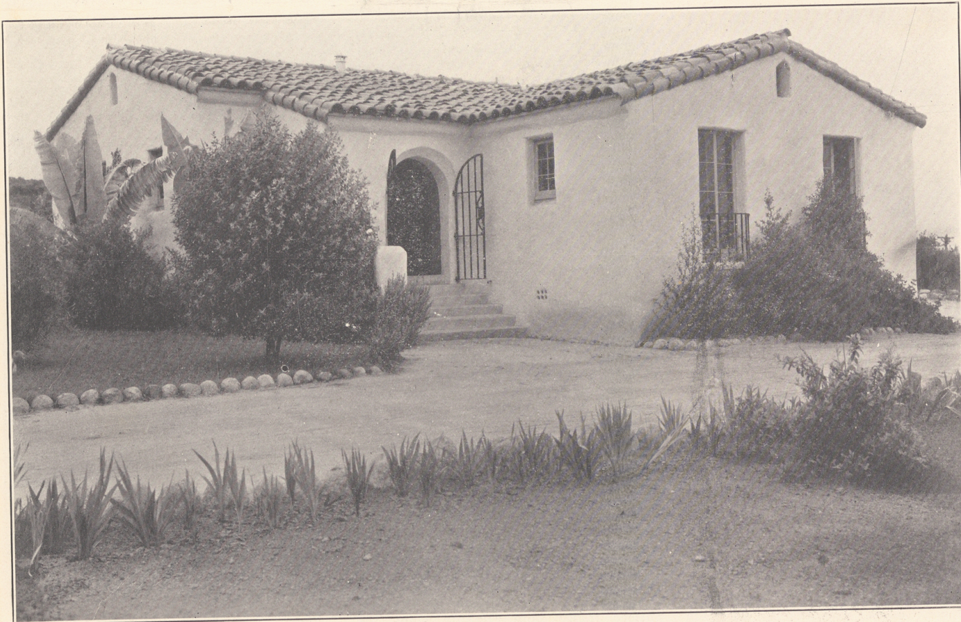
Santa Fe Irrigation District headquarters at Rancho Santa Fe. Architecture conforms to the prevailing Spanish type.
