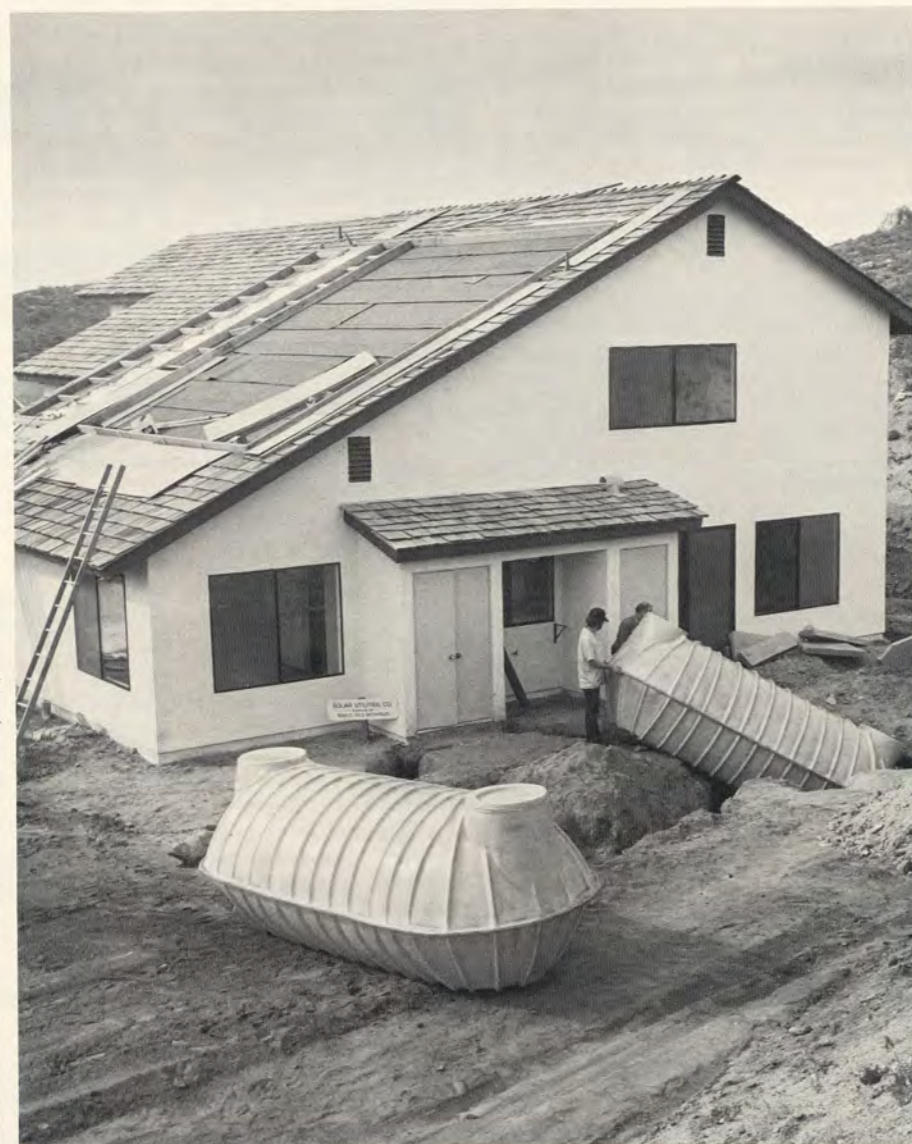
Two 1,500-gallon resin-reinforced fiberglass storage tanks at SDG&E's solar demonstration house. Photo courtesy SDG&E.
