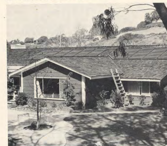
Fafco pool heating units on the roof of the Dempsey home. Note how well units blend into roof. Photo by Donnelly.
