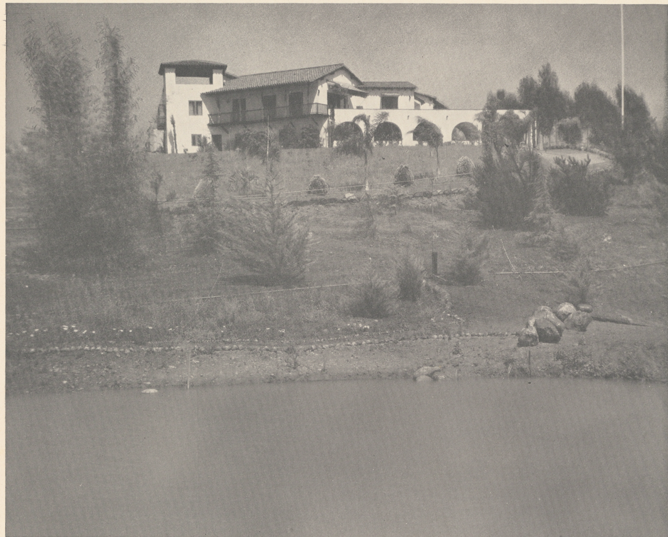
The C. F. Pease home is one of the most impressive at Rancho Santa Fe. A little lake, a winding drive, rolling ground above the river and extensive landscaping make this estate truly attractive.
