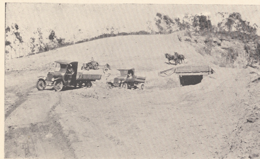
Trucks, teams and men getting surface material for the new roads in Del Bosque.
