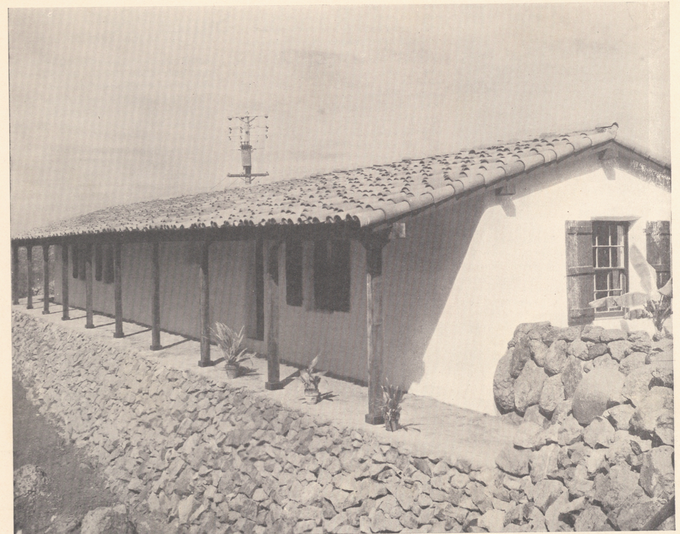
The beauty of the pump-house on the Fairbanks estate speaks volumes for what may be expected when this great development is completed.
