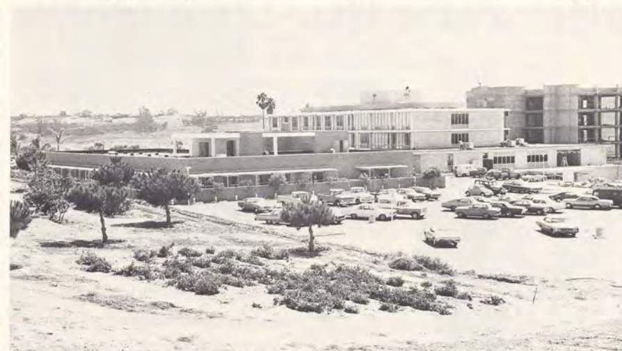
Who wouldn't be excited! The low structure on the left is the new extended care unit just completed — and on the right the new tower building is already taking shape.
