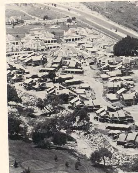
The final 54 units in San Vicente Country Villas II, a $6,600,000, 110-unit condominium complex, are scheduled for completion in July. The complex is adjacent to the San Vicente Country Club golf course at San Diego Country Estates, a 3,200-acre resort community located 44 miles northeast of San Diego.
