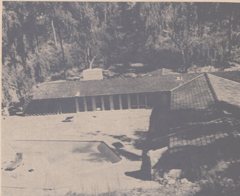
POOL INCLUDED — Under construction is home of Mrs. Ruth L. Swisher.
