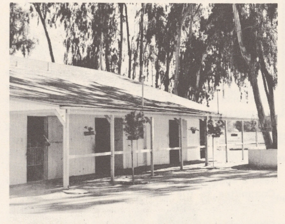
Each stall at Pasatiempo has an iron stall guard so top and bottom doors can be left open for better ventilation. Automatic watering has been installed in each stall and paddock providing the horses with continual fresh, clean water.
