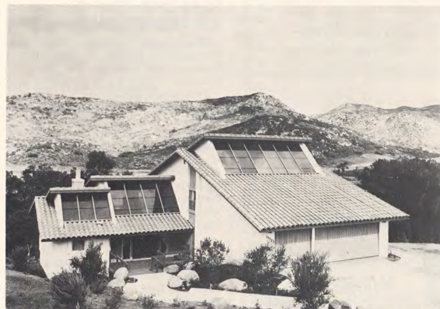
Solar panels of "Vicente del Sol," one of the first homes in Southern California to utilize solar energy for its heat and hot water, are incorporated into the roof design as architectural features resembling skylights.
