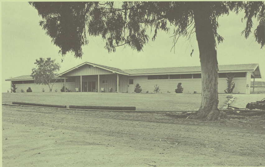
The front view of the new horse barn at Ranchito Allegre. The office section is in the center of the barn.
