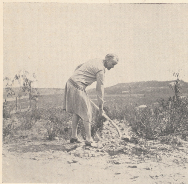
Mrs. Ellis Bishop breaking ground for the Bishop home on a picturesque ridge in Block 36.
