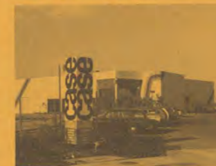
Case warehouse, east elevation
