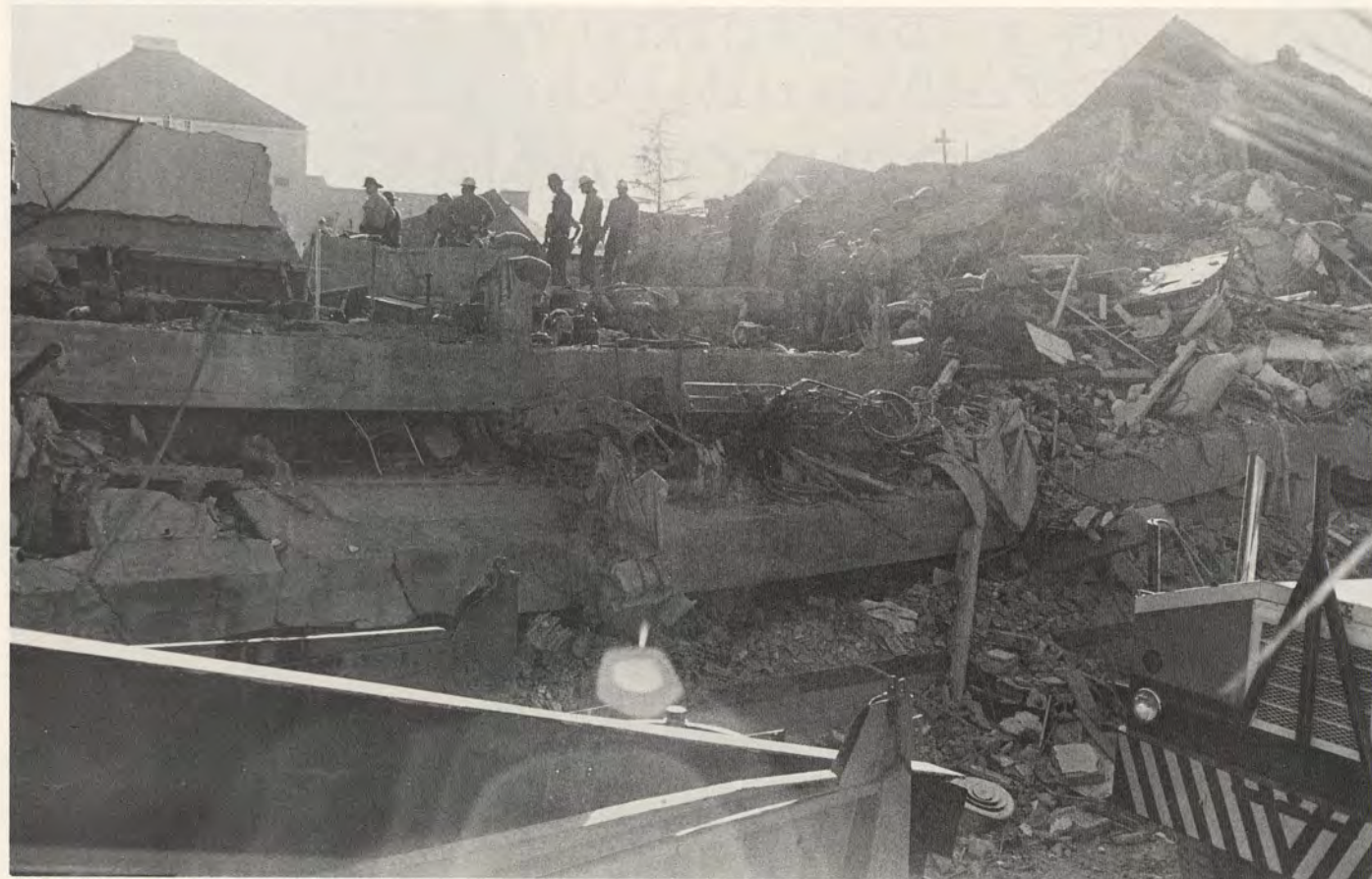
The Sylmar Veteran's Hospital, an older structure built of unreinforced masonite, was reduced to rubble. The hospital was a four-story structure and in this picture, three of the four levels are visible. The fourth is underground.
