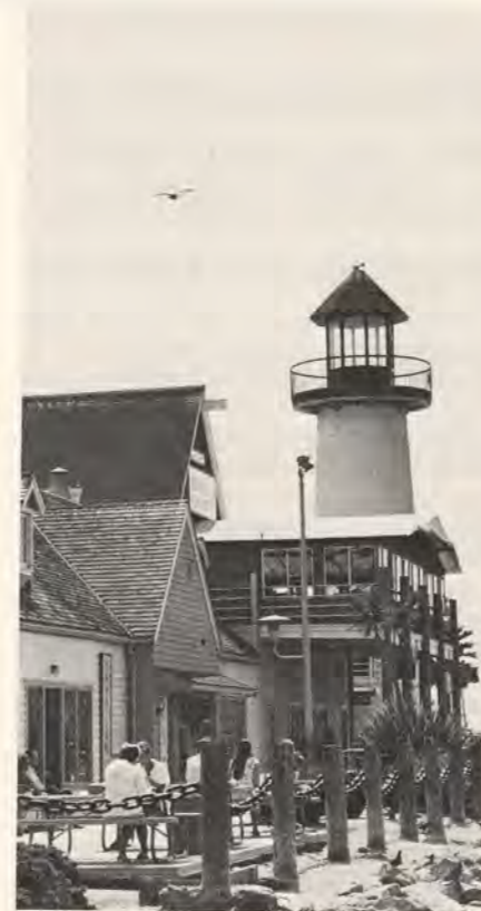
Cape Cod Village, the main shopping area for the Oceanside Small Boat Harbor. Restaurants, a few stores and marine parts and repair shops are the major attractions. The structure jutting out directly in front of the lighthouse, which is mostly decorative, but does house a boat broker in its base, is the Mainsail Restaurant.
