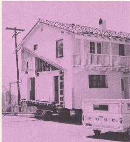
Smooth sailing once more at the intersection of Linea del Cielo and Las Flores. Only a few leaves were pulled off the trees because of the skill of the movers crew.
