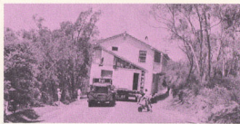
Ob, ob! Trouble on the sharply banked curve between La Glorieta and El Cielito. Because of the steep angle of the curve the weight shifted precariously and bent the heavy steel beam supporting the rear end.
