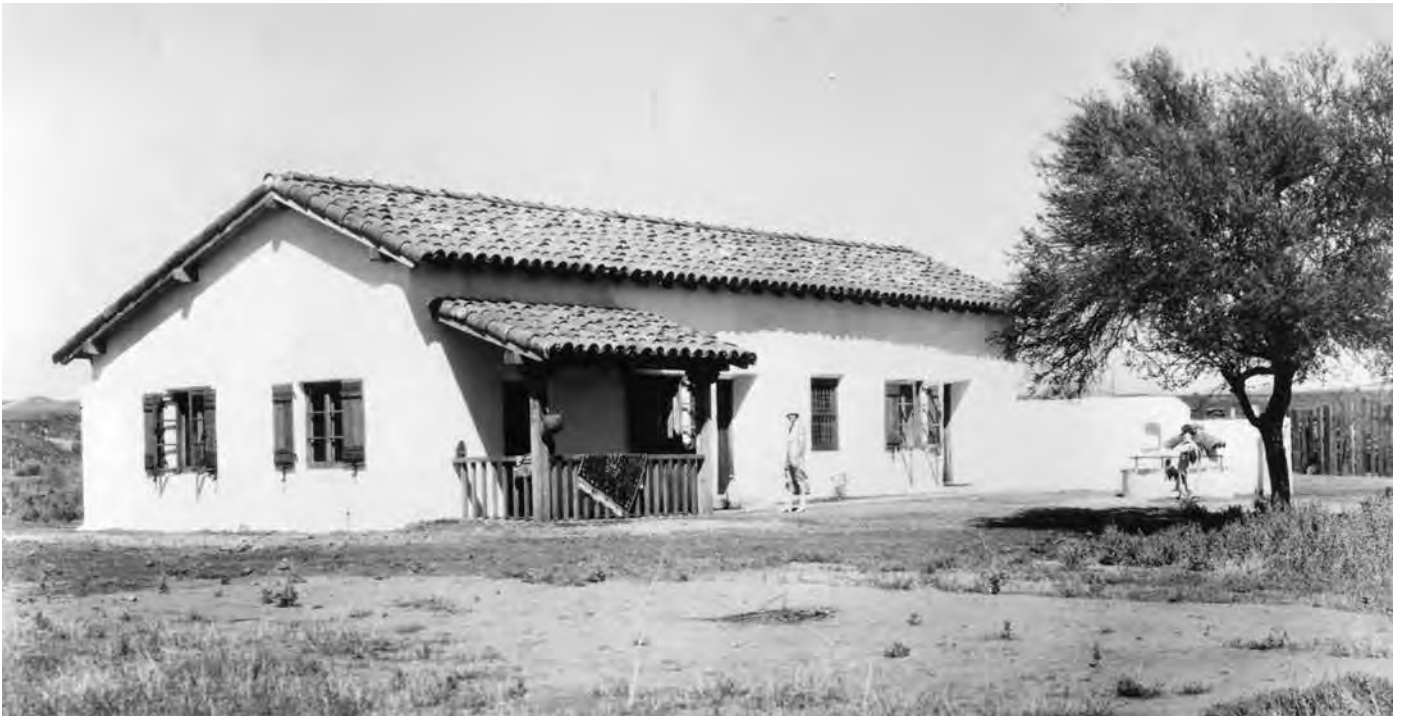
Figure 2.7 Completed Rehabilitation of Osuna Adobe #1
