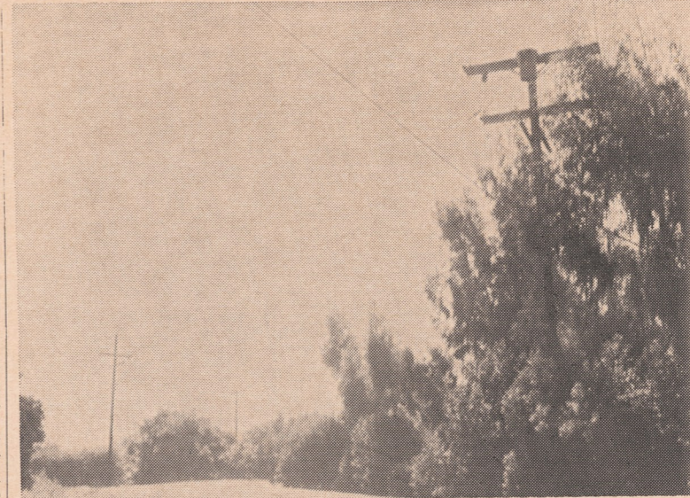
CAMOUFLAGE PROBLEM — This photograph of a telephone pole on the Ranch illustrates what can be done with a little planting. It should be placed far enough away from the pole to permit maintenance of the lines, but close enough to obscure the harsh vertical pattern of the structure.
